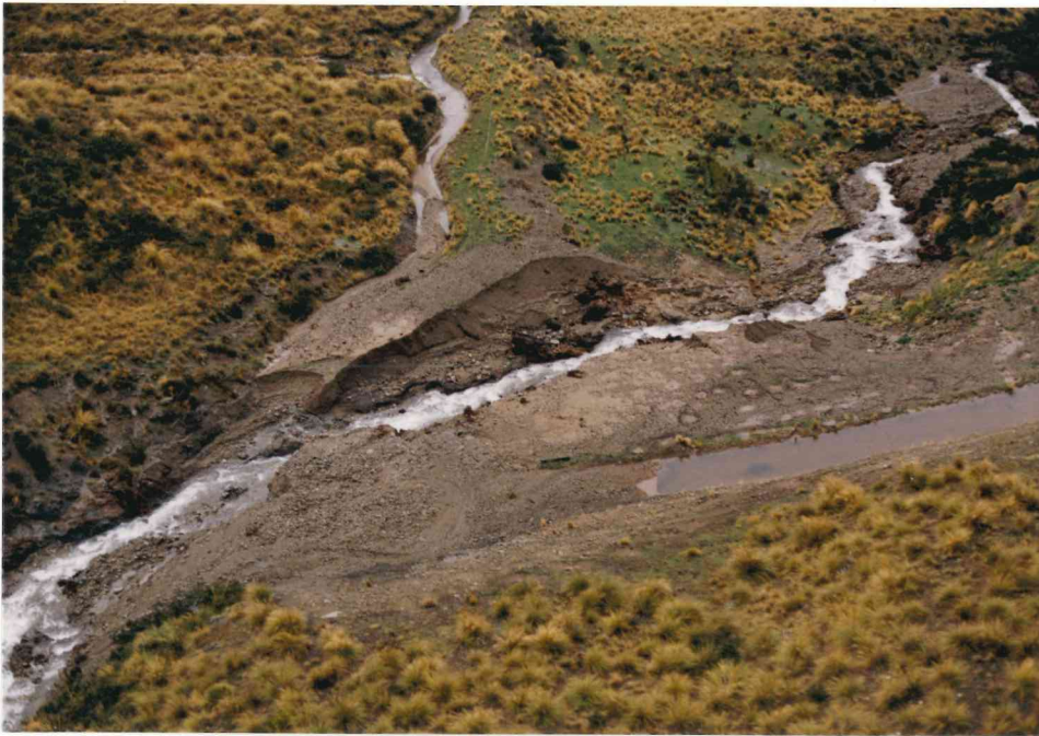
Photograph highlighting damage to the Mount Ida race at Little Ten Chain Creek
