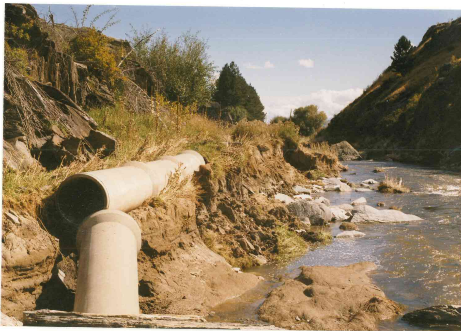
The above photograph highlights the extent of damage to the Idaburn Intake
