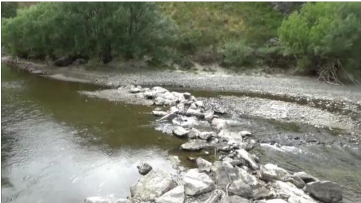
Figure 49. Manuherikia Scheme intake 11 th February 2019. Daily average flow at Campground 0.693 m 3 /s.
