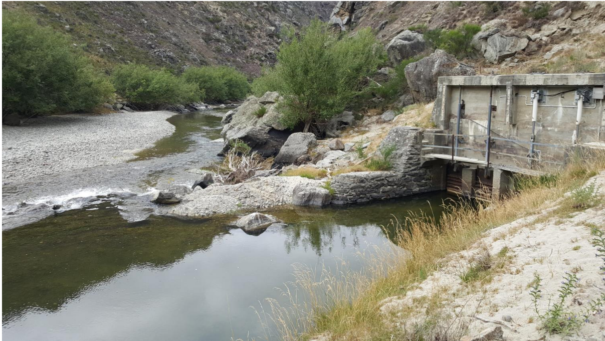
Figure 8. Looking downstream at the MICS intake
