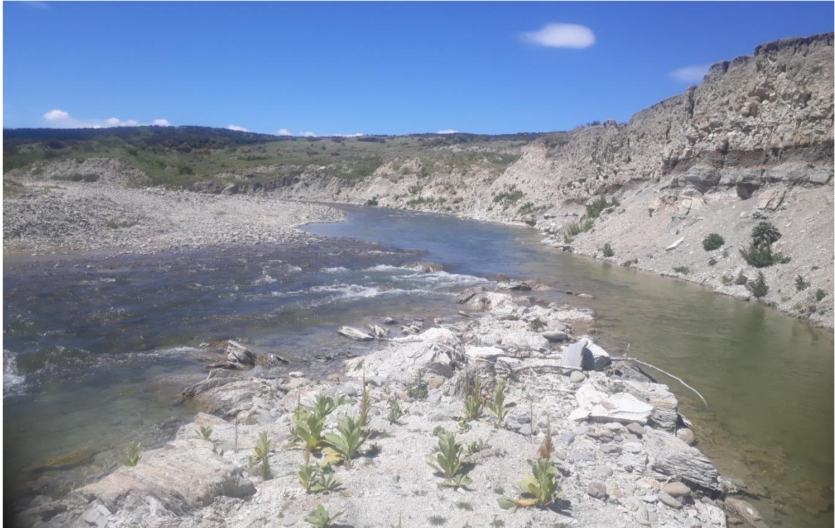
Figure 45. Blackstone irrigation Company intake.
