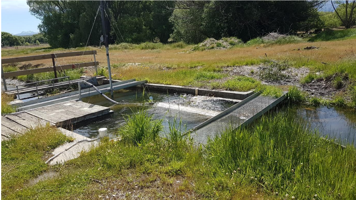
Figure 52. Intake and Screen at the GIS pumps.
