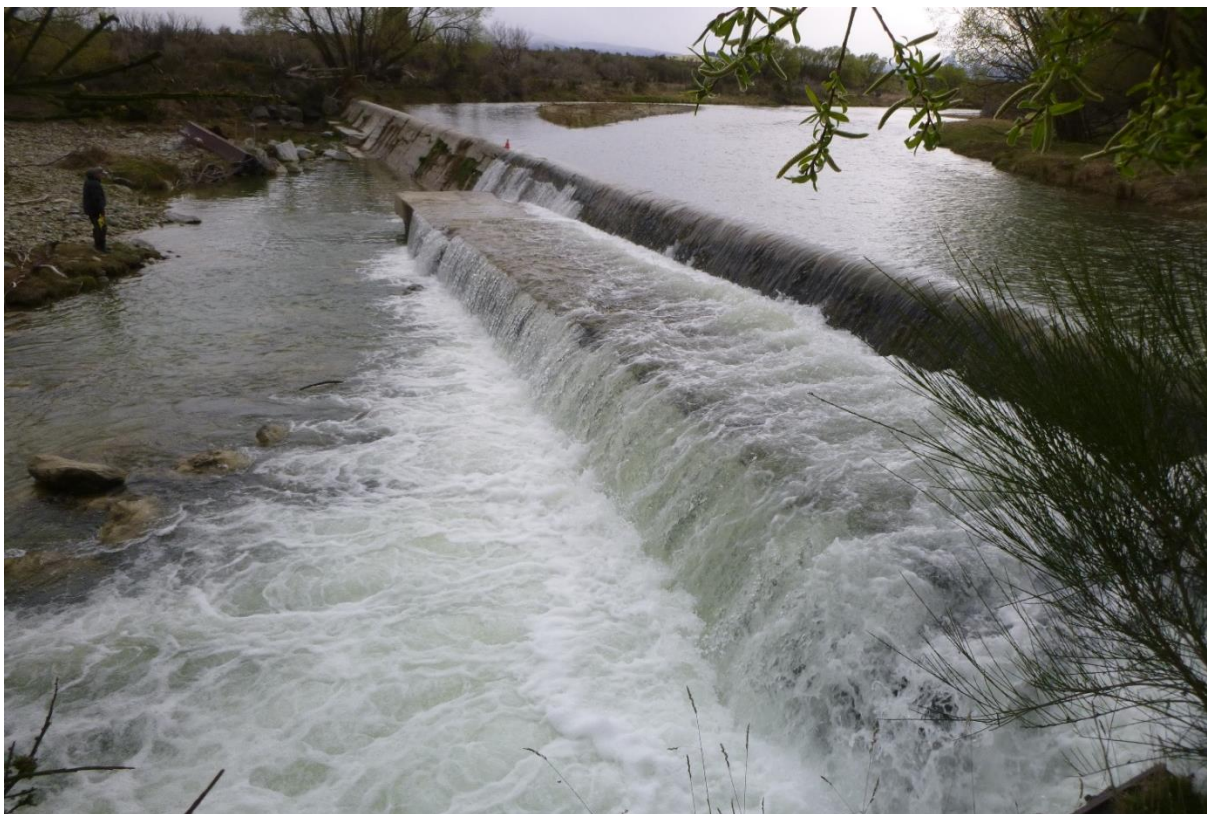
Figure 48. Photograph of the OAIC main race intake on the Manuherikia River from the True Left bank.
