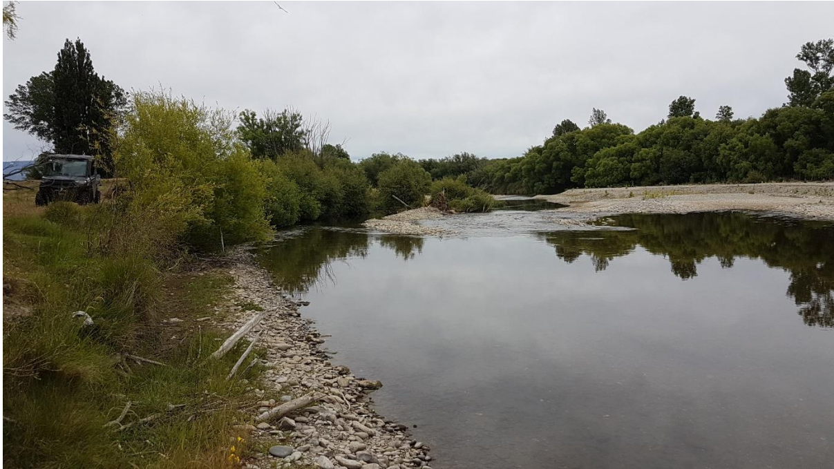
Figure 50. GIS intake with a flow of approximately 1.6 m 3 /s Campground.
