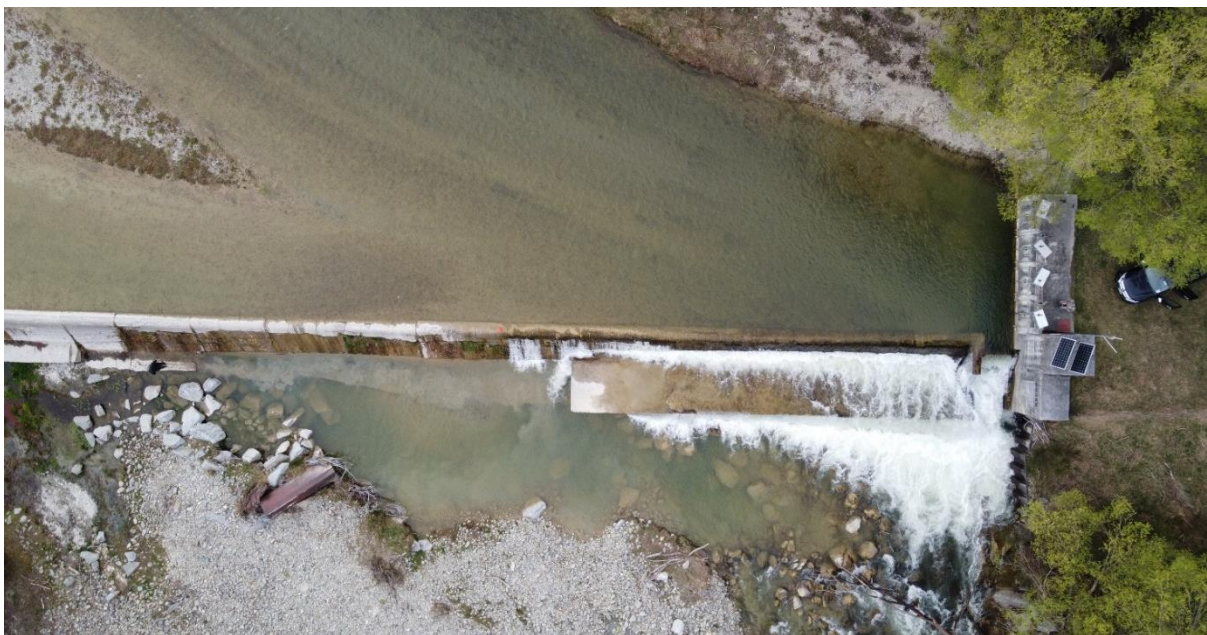
Figure 46. Aerial Photograph of the OAIC main race intake on the Manuherikia River.
