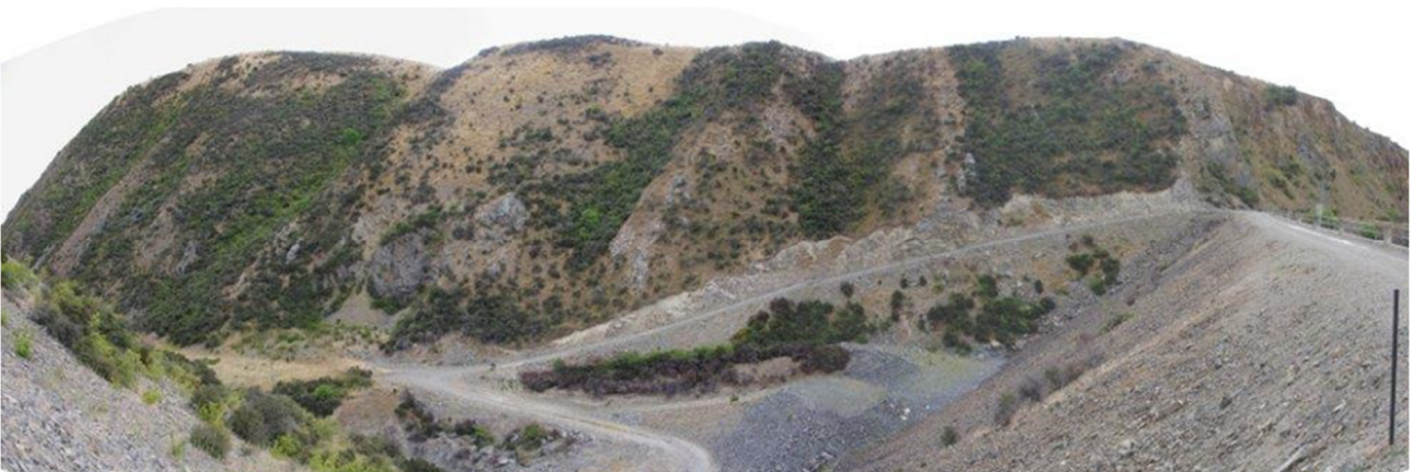
Figure 9 Wide angle view of right abutment area
