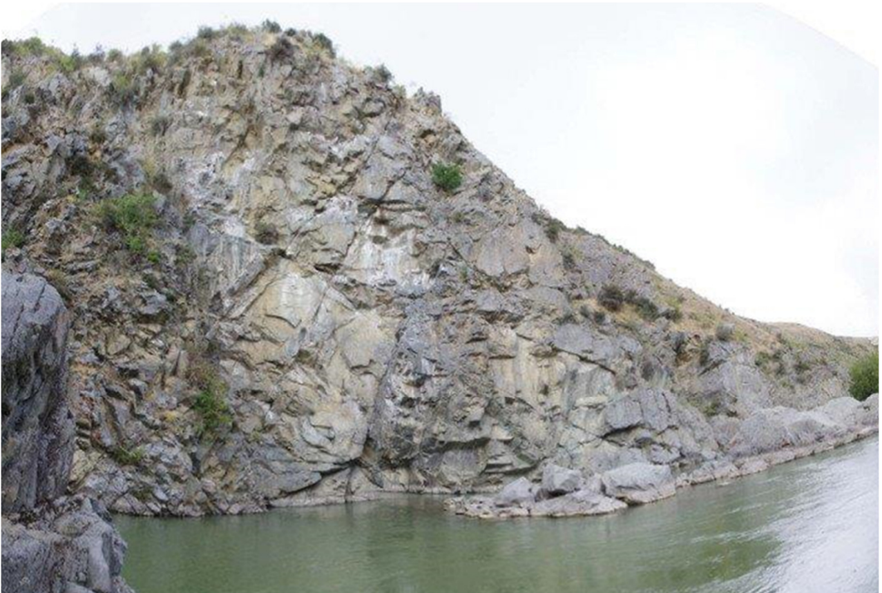
Figure 11 View of steep rock mass exposure on left bank of river near proposed spillway chute
