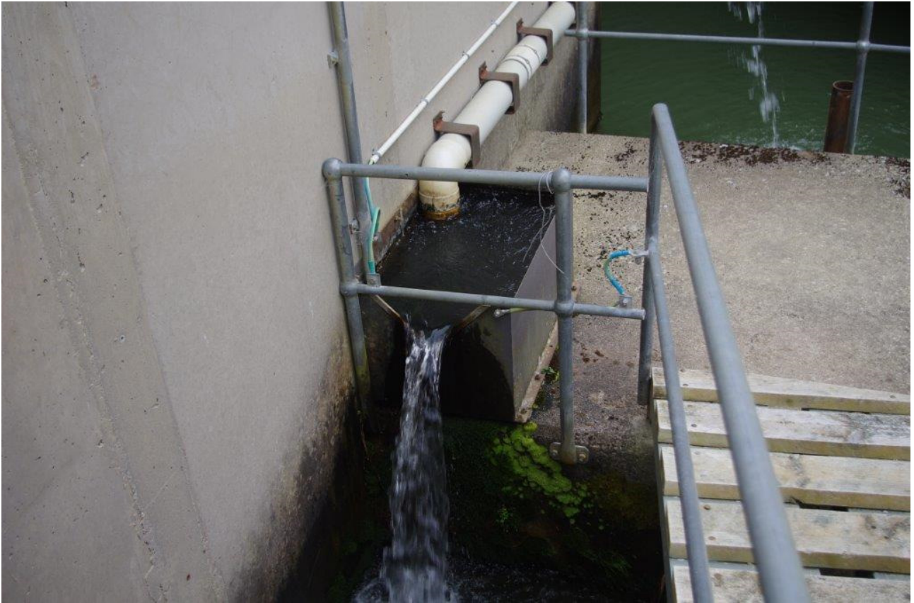
Figure 21 Seepage monitoring prior to c2015 membrane repair (115mm on V notch)
