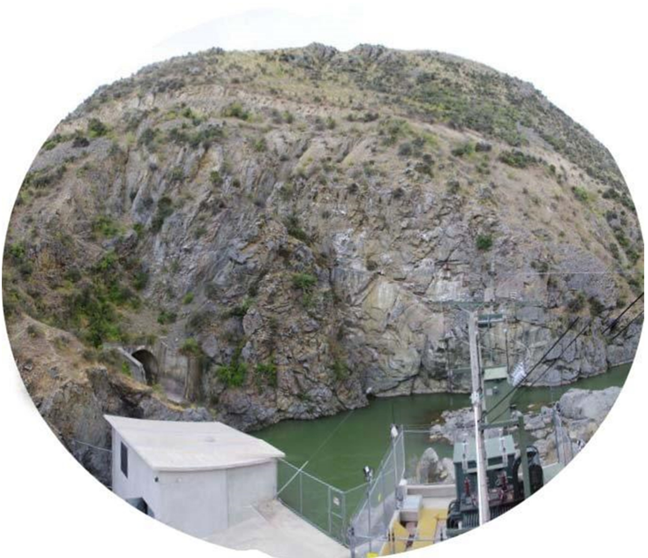
Figure 10 View of rock mass exposure downstream of tunnel portal
