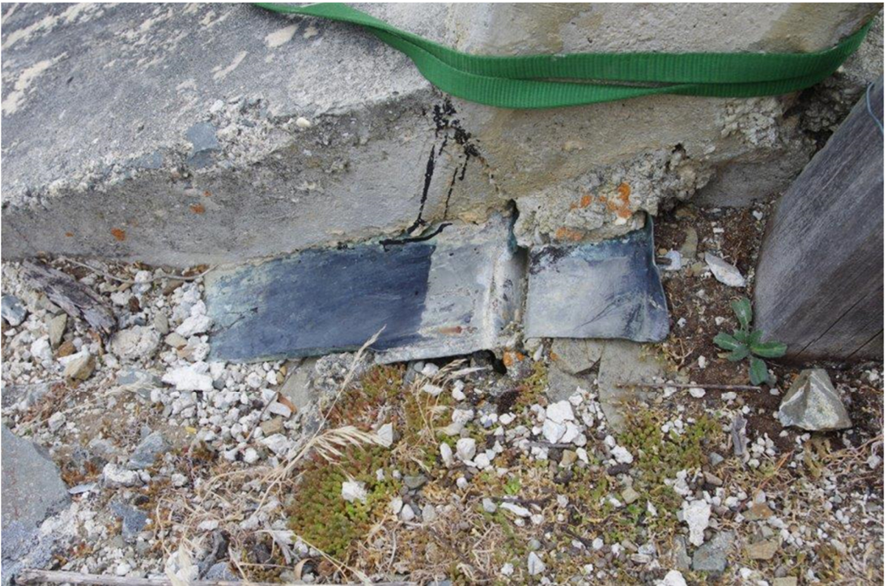
Figure 22 View of Cu waterstop exposed at TR crest c2015
