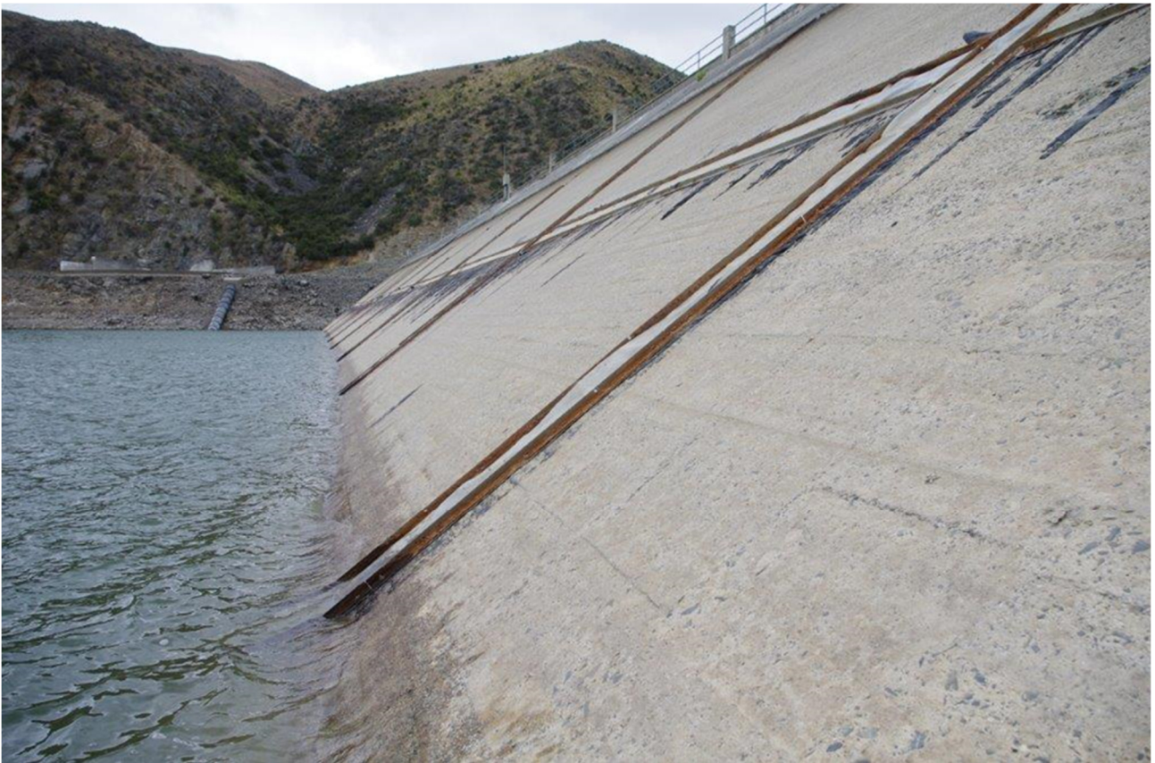
Figure 19 c2015 view of membrane
