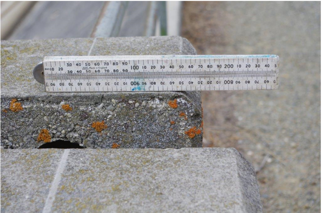
Figure 15 Offset at TR double post c2015
