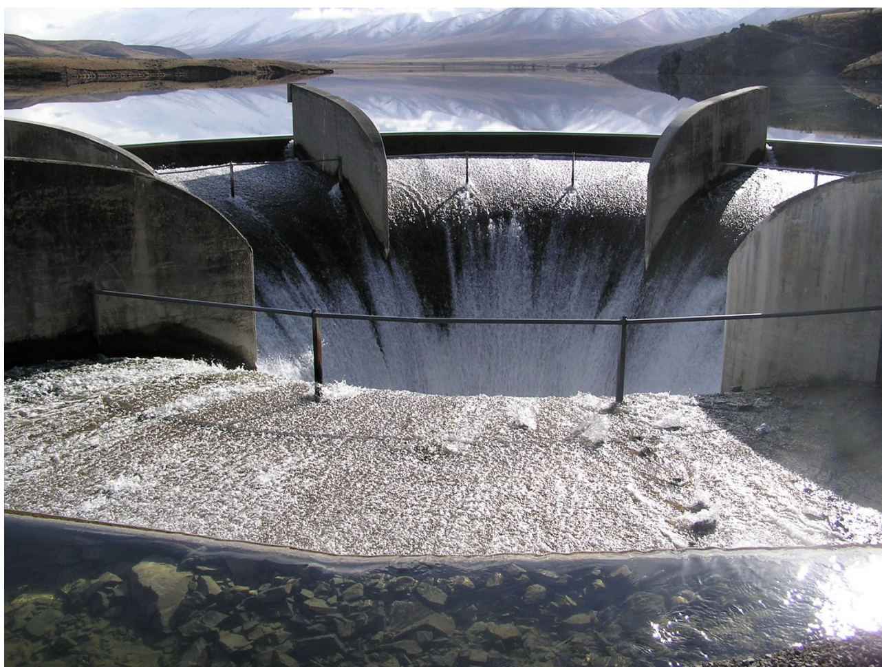
Figure 3 bell mouth spillway showing raised sill
