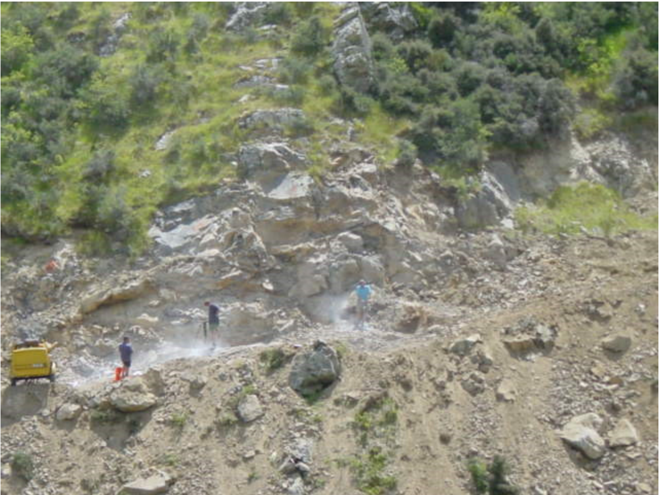
Figure 8 Excavation for hydropower scheme c2003 illustrating typically limited surficial cover
