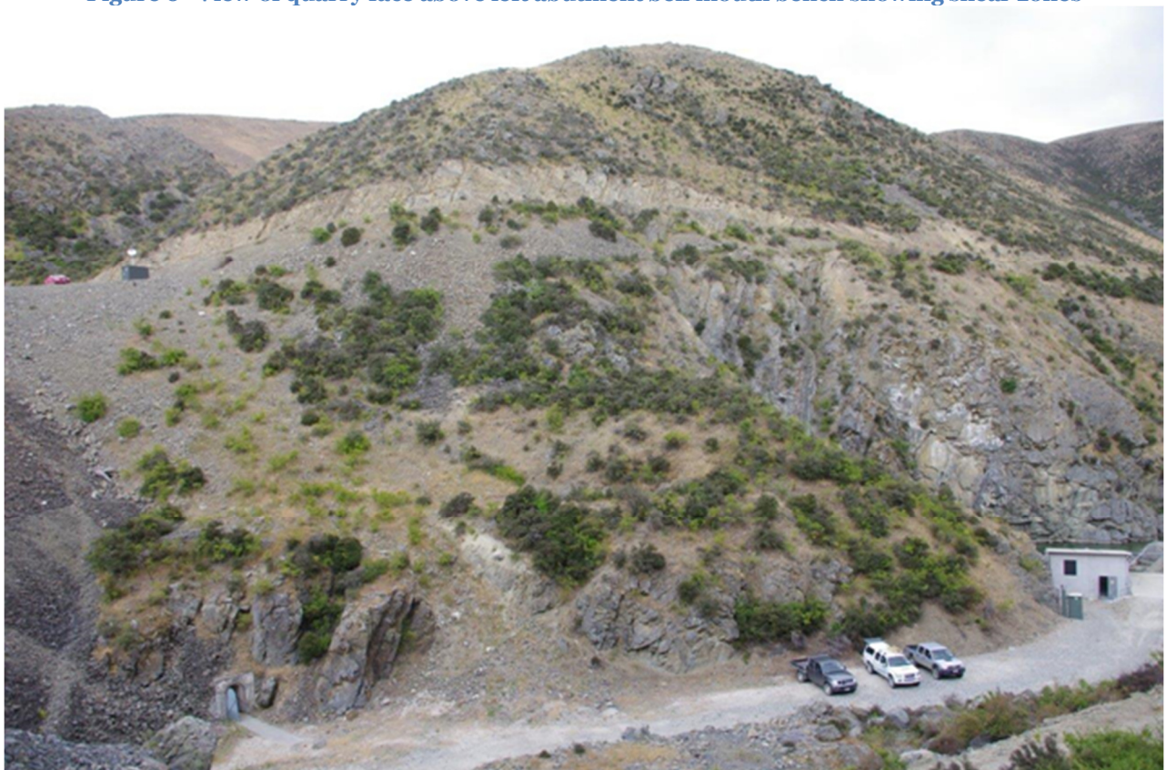
Figure 7 View of Left Abutment. Valve chamber access adit at lower left, Powerhouse Lower right.
