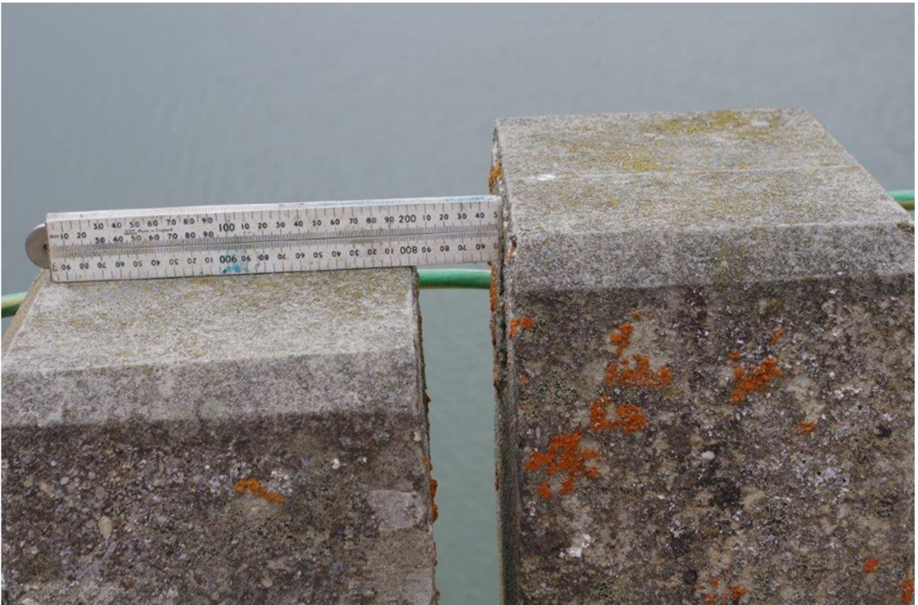
Figure 16 Offset at TR double post c2015
