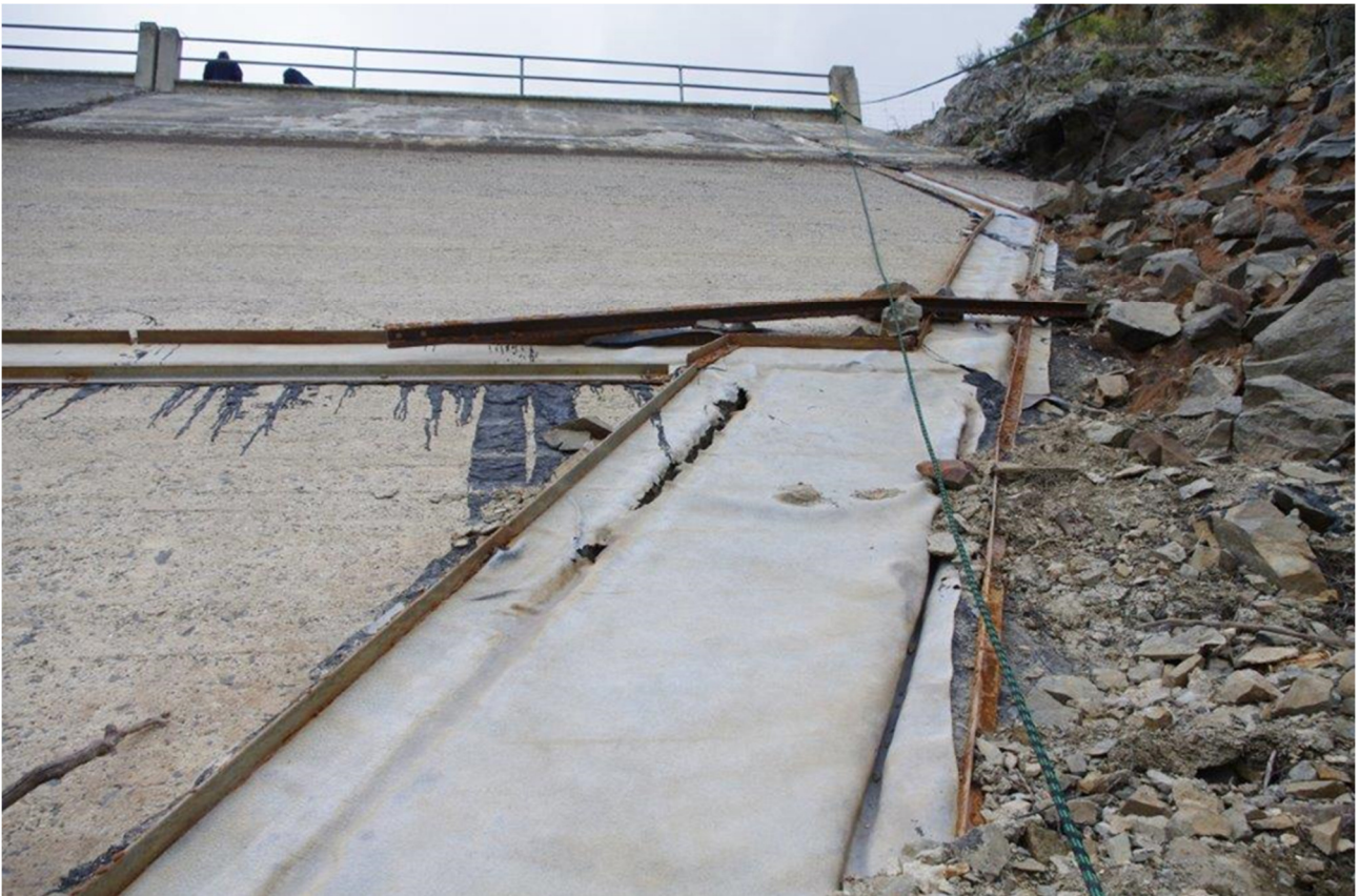
Figure 20 View of TR perimetric joint prior to 2015 repair
