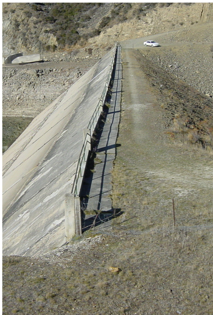
Figure 13 View of crest settlement c2001
