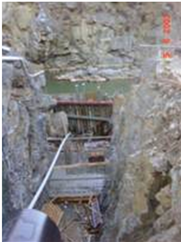
Figure 12 Excavation for Powerhouse at original falls
