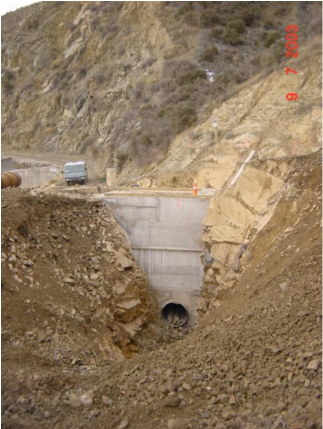
Figure 24 DN1200 Penstock Cut Off at Crest
