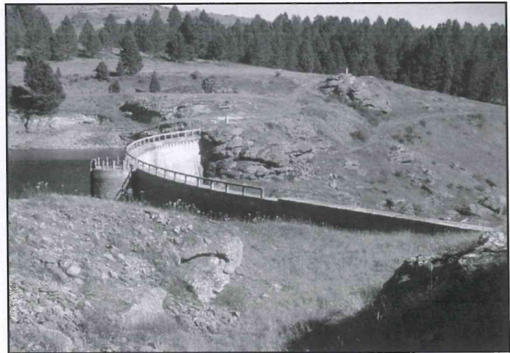
A recent view from the location where the cableway operated. Above the left abutment can be seen the platform for the rail track, which allowed the cable to span the main part of the dam.
