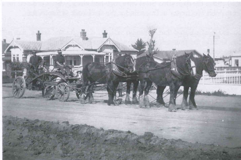
An early road grader working in a street at Christchurch. This would have been similar to the road grader which was used on the road up to the Upper Manorburn Dam site. These graders were made by Caterpillar and required an operator at the rear who controlled the blade and a second person who handled the horses.
