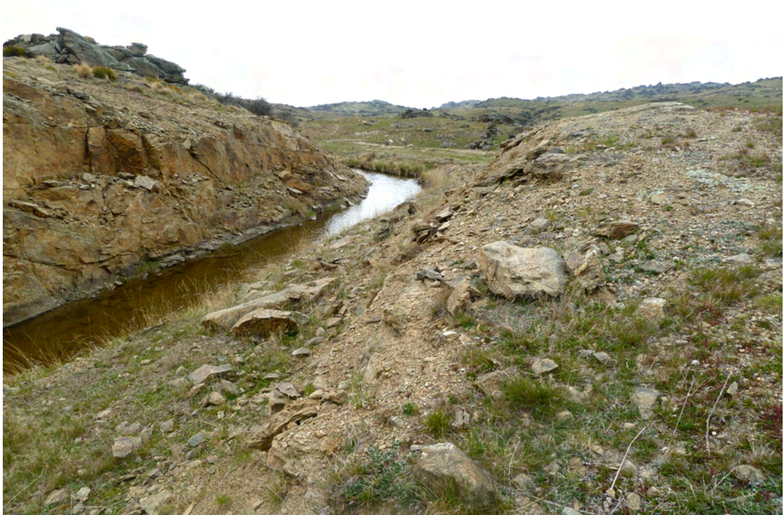
Figure 3.8: Upper Bonanza Race just upstream of where the proposed syphon would join. The race has been relocated through a low saddle. Photo looking south 24 Oct 2012
