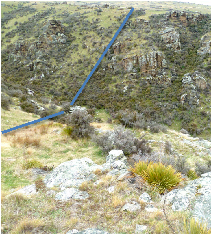
Figure 3.7: Syphon route through Manor Burn valley from part way down slope below Upper Bonanza Race looking SW to left bank. Syphon would start mid photo nearer ridgeline. Indicative alignment is shown (Photo 24 Oct 2012)
