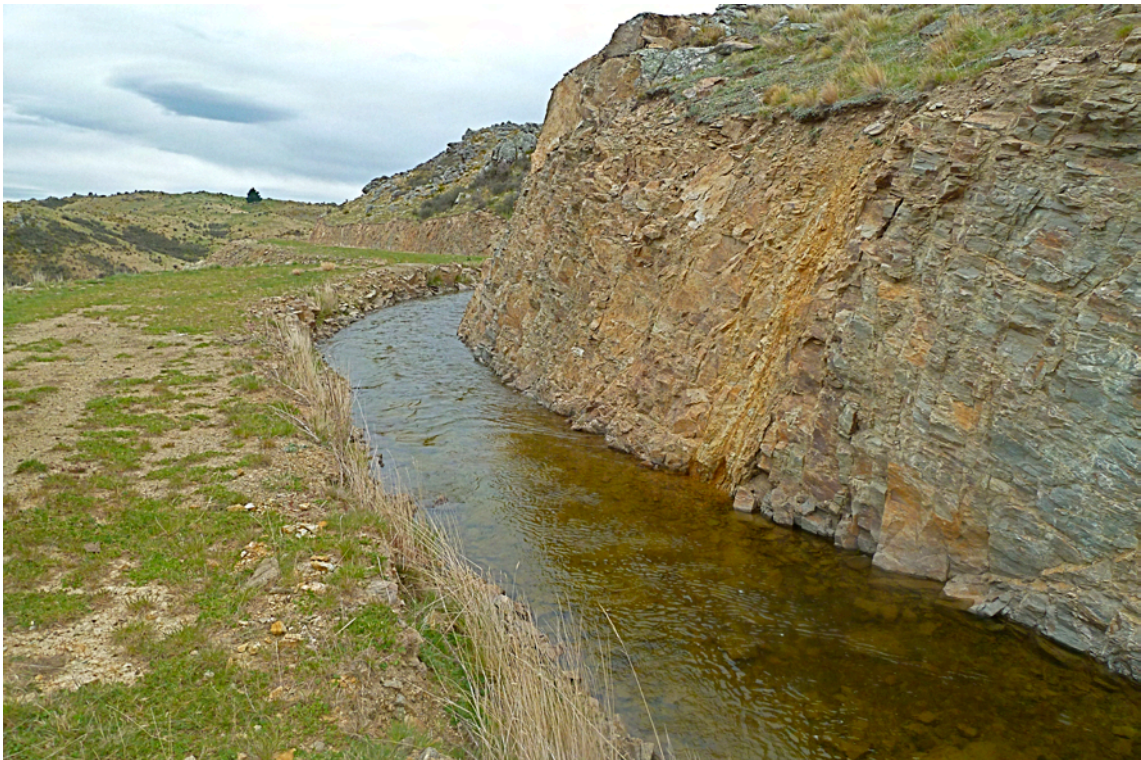
Figure 3.4: Upper Bonanza Race close to site where Hopes Ck Diversion Race would enter. Similar country is expected in parts of the diversion race (Photo 24 Oct 2012)
