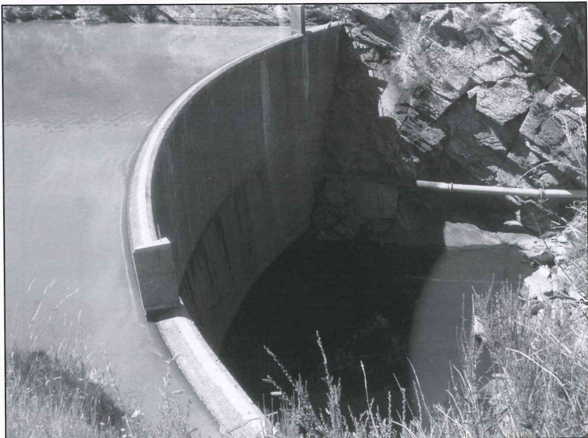
A recent photograph taken above the right abutment. The shaped crest can be seen with two splitters to improve the water discharge during floods. The pipeline is visible on the left side of the stream, tucked under the downstream cliffs. A natural pool has been formed downstream of the spillway by the flood discharge.
