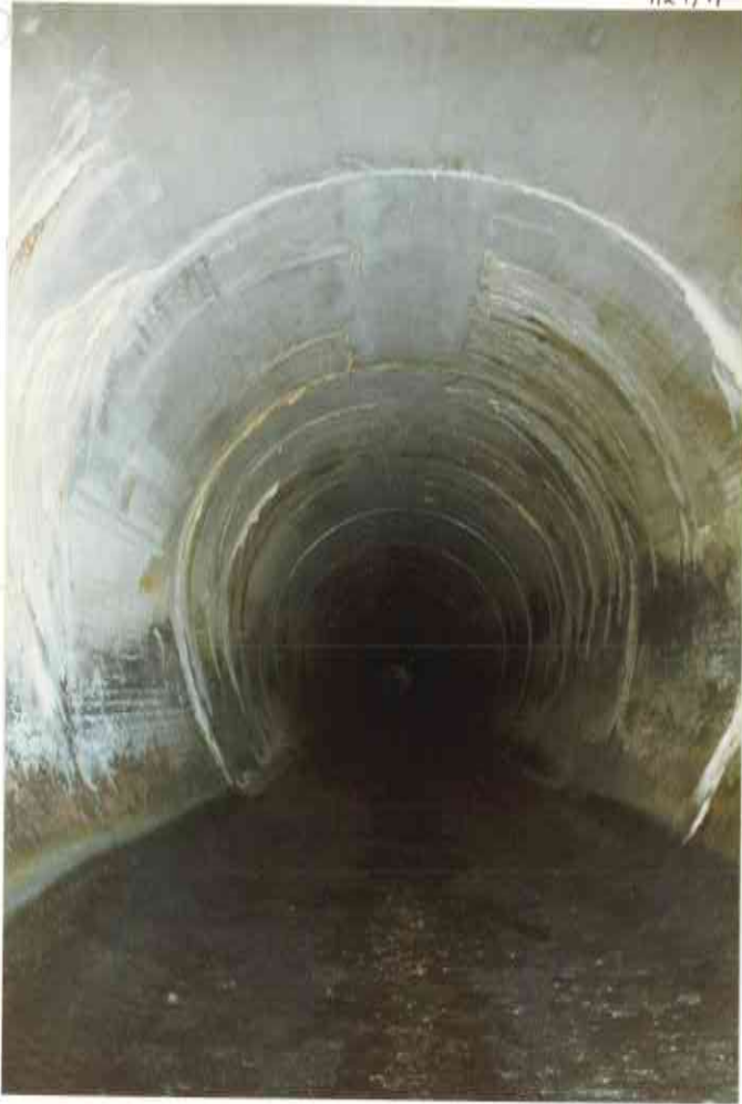
15. TYPICAL OF TUNNEL VIEWED U/S
