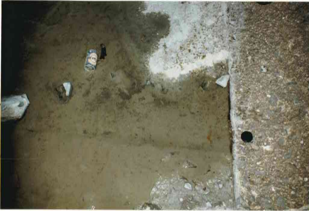
24. JT 31/32 AT INVERT VIEWED D/S
