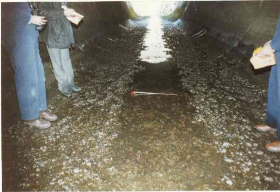
7. TYPICAL OF INVERT, 27" OF TAPE SHOWING
