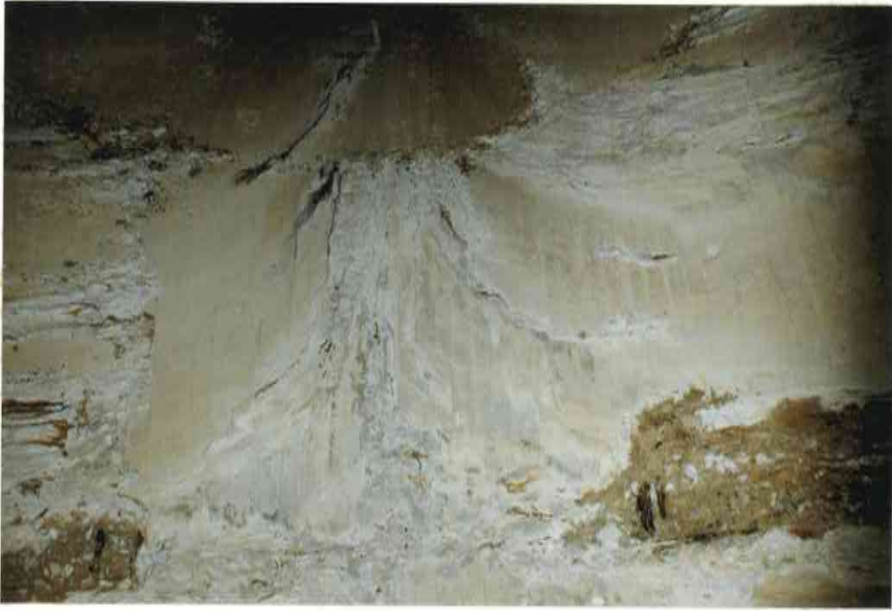
26. CROWN OF PANEL 32 SHOWING STEEL EXPOSURE AT JT 31/32 AT BOTTOM
