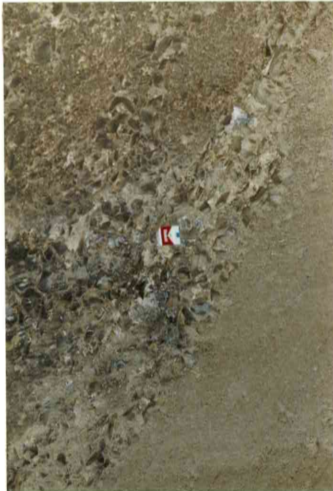
26. CROWN OF PANEL 32 SHOWING STEEL EXPOSURE AT JT 31/32 AT BOTTOM
