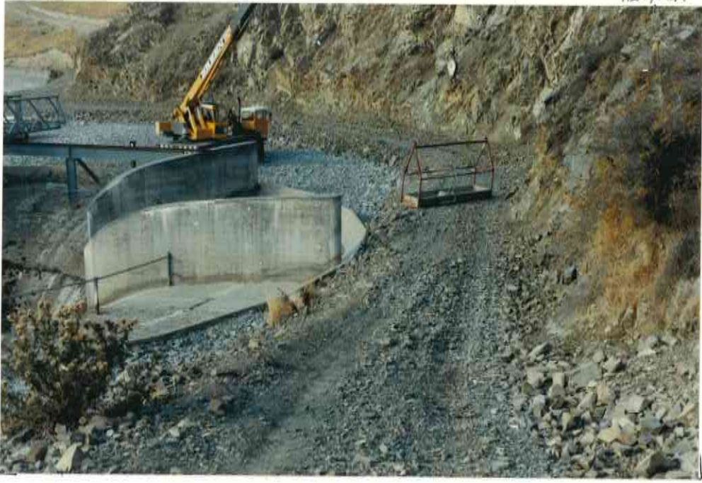
88. ACCESS TRACK PASSED SPILLWAY
