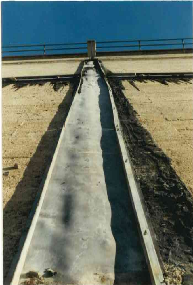
96. VERTICAL JOINT BETWEEN THE SECOND AND THIRD PANELS
