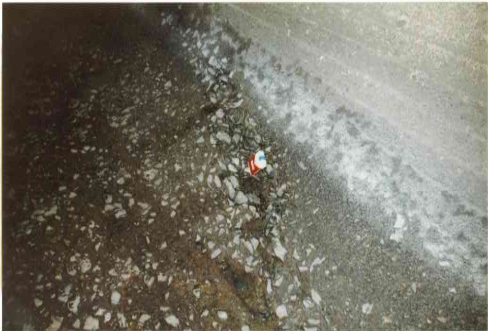
10. I/W jt TR, EROSIAN 130mm DEEP, 200mm WIDE 1.1m LONG
