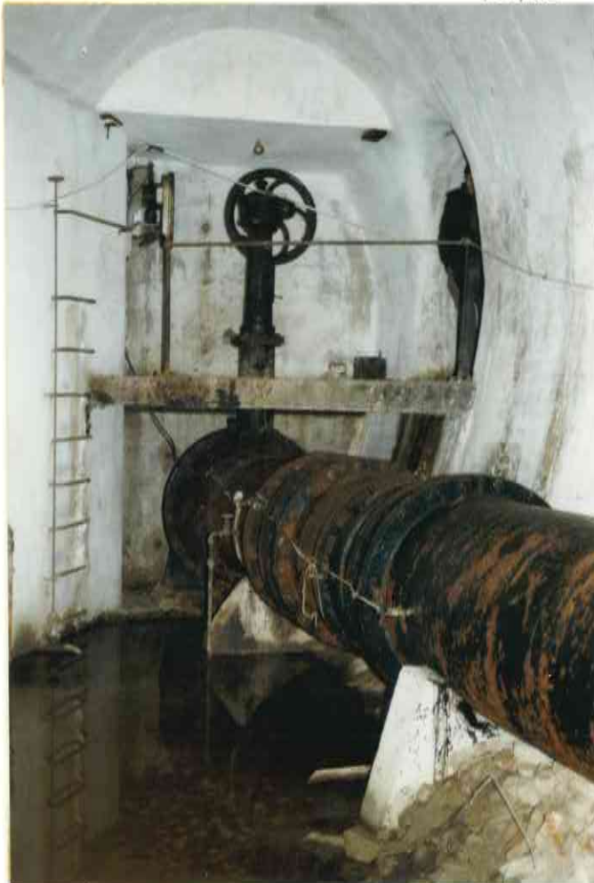
2. NEEDLE VALVE CASING & GEARS
