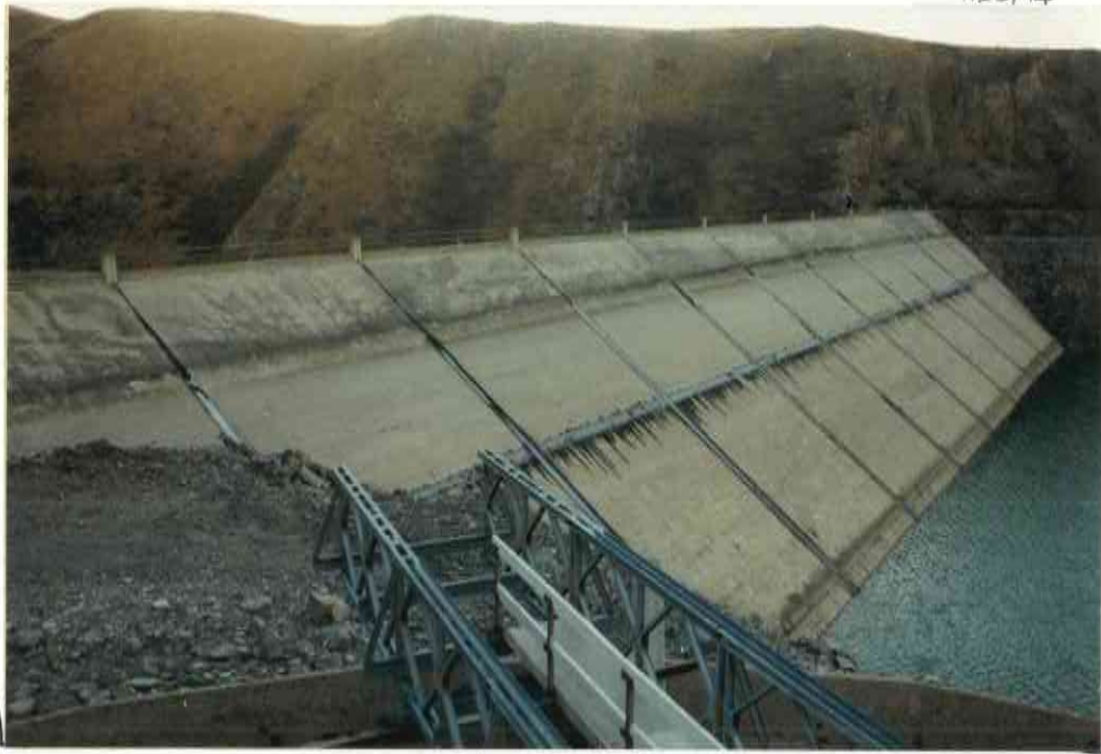
90. DAM MEMBRANE VIEWED FROM ABOVE
