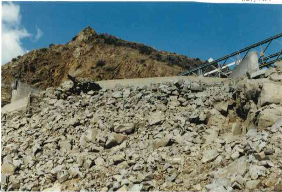
87. LOOSE ROCK SLOPE BELOW BAY 5, IN SITU ROCK TOP LEFT + TOP RIGHT
