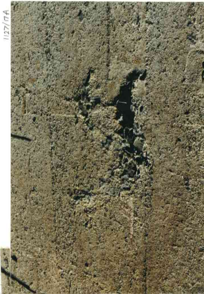
92. CONCRETE SURFACE DAMAGE NEAR THE ABUTMENT MIDWAY DOWN SECOND HORIZONTAL PANEL ROW
