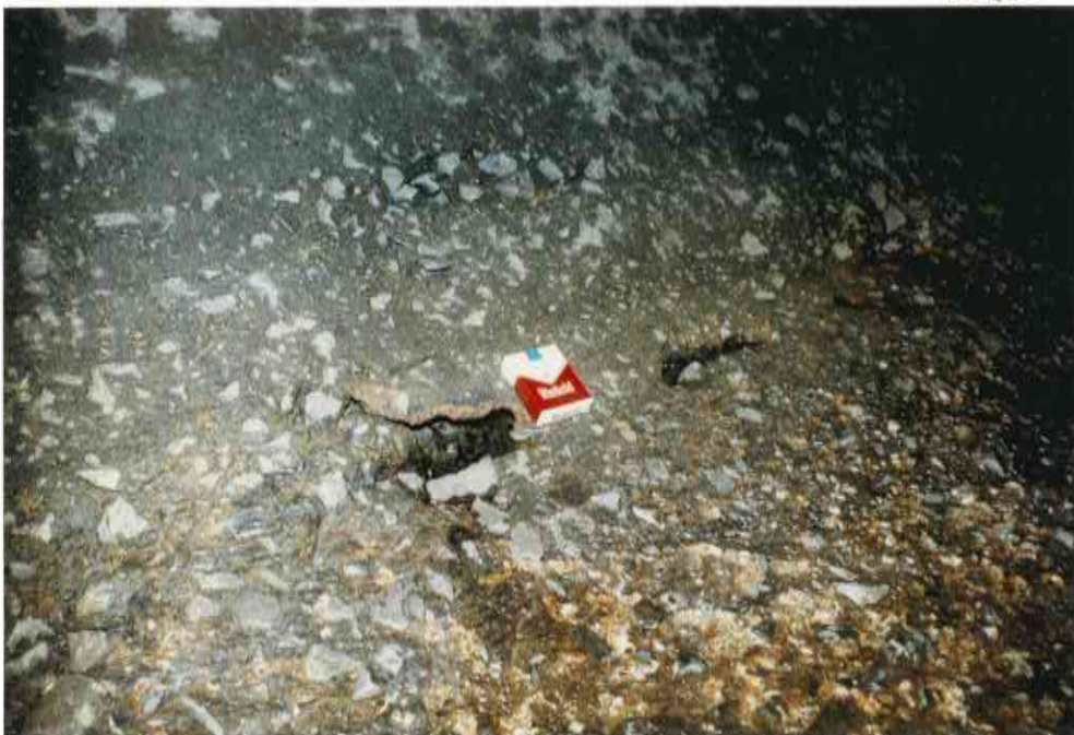
16. CAVITY UNDER WALL TL I/W jt
