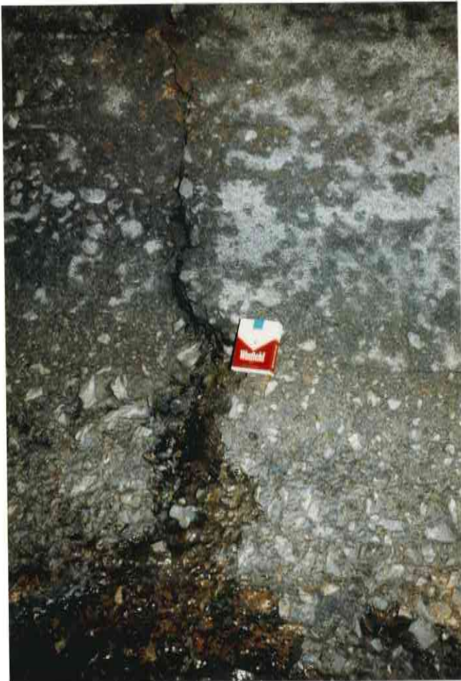
14. TYPICAL OPEN JOINT (Jt 16/17) BETWEEN PANELS
