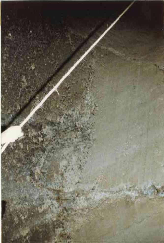
28. TL MID-HEIGHT CONSTRUCTION jt
