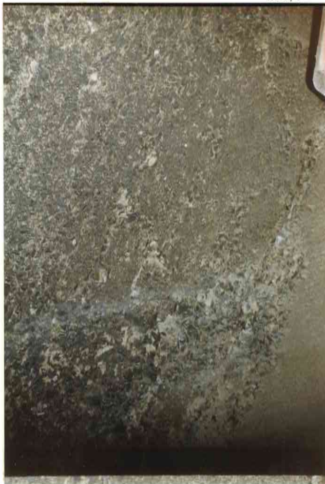
29. TL MID-HEIGHT CONSTRUCTION jt
