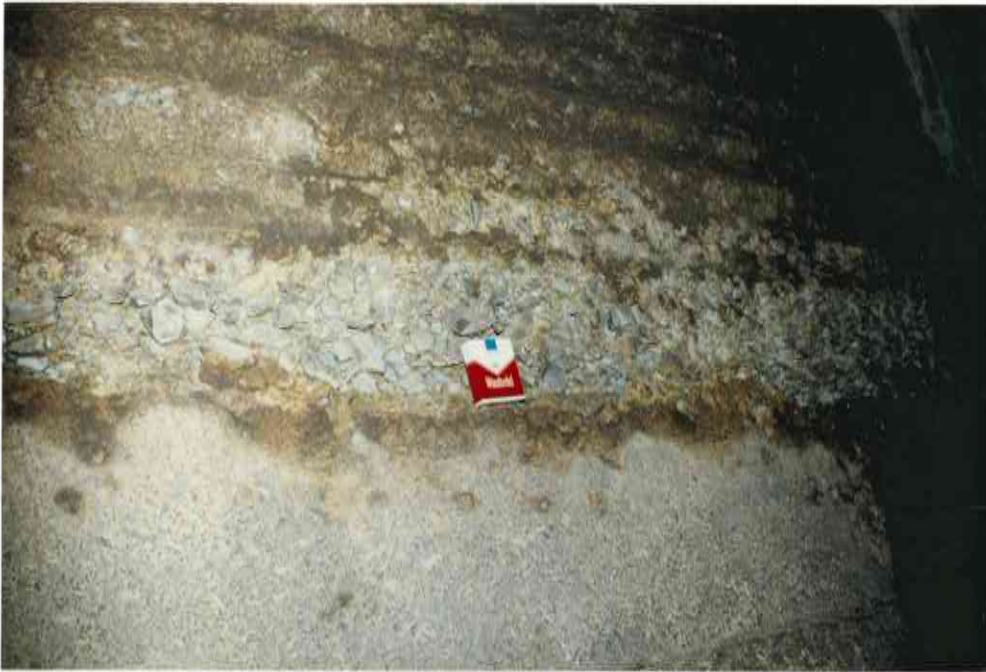
13. HOR jt 1.5m ABOVE INVERT TL FULL LENGTH POLYMER 200mm HIGH + 80mm DEEP
