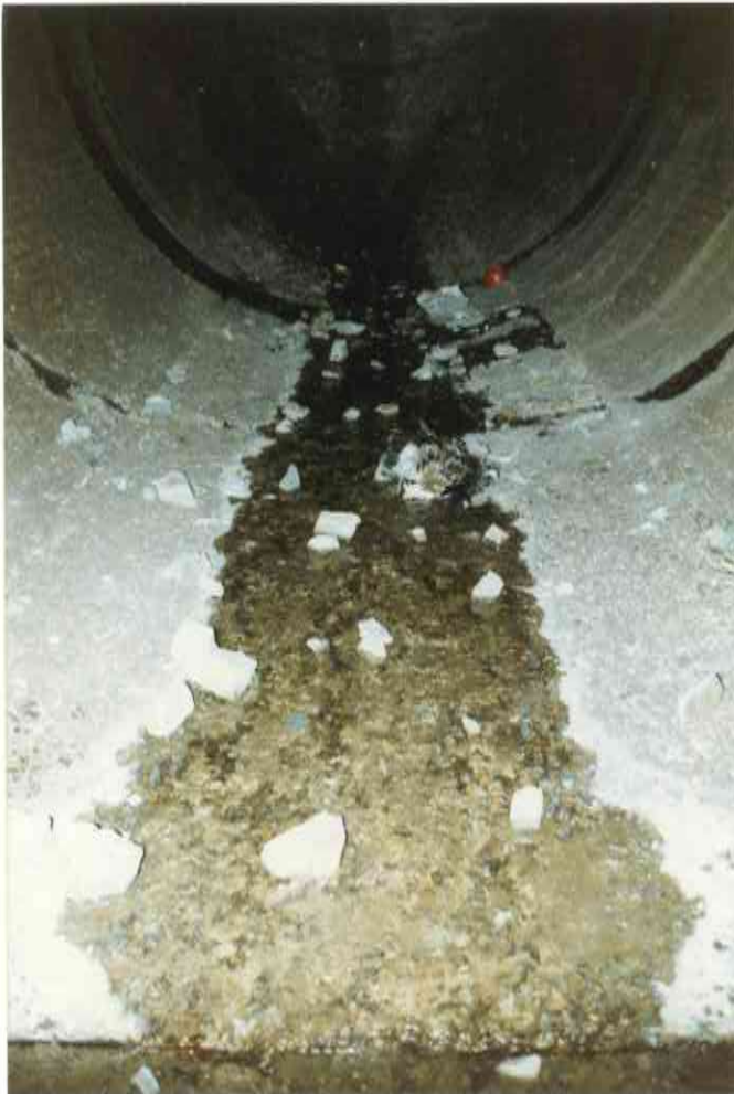
23. PANEL 30 INVERT LOOKING U/S
