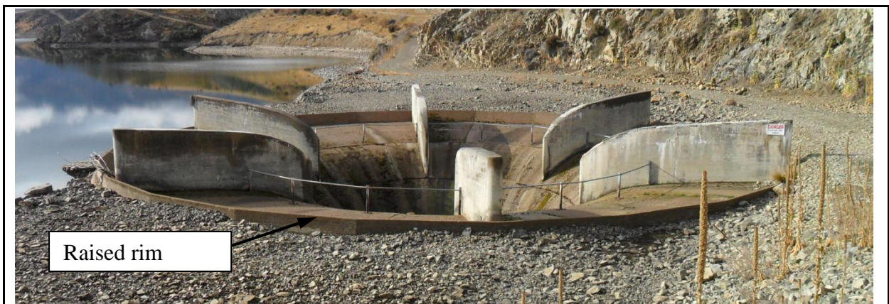
Current spillway with raised rim
