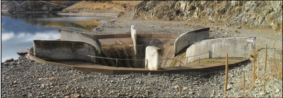
Figure 13: Morning Glory spillway
