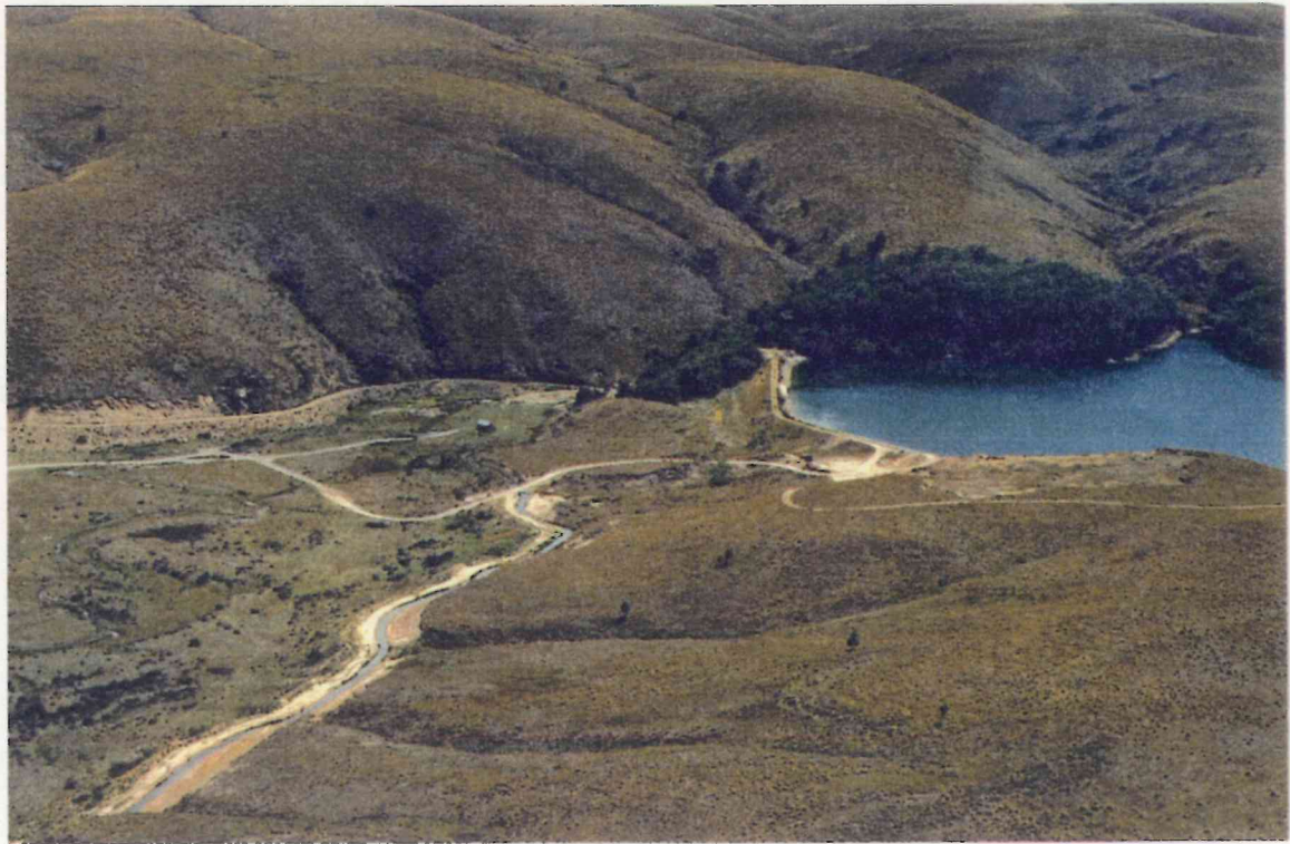
West Eweburn Dam January 1990
