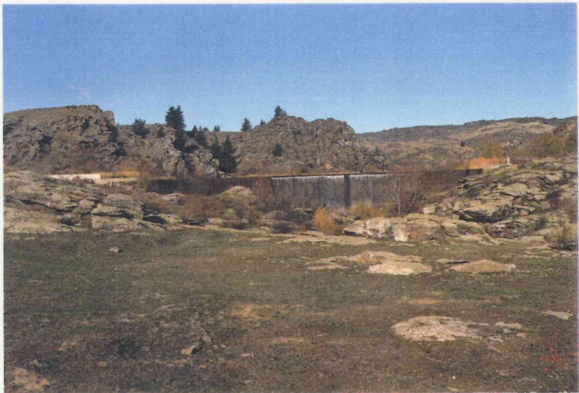
Lower Manorburn Dam May 1990
