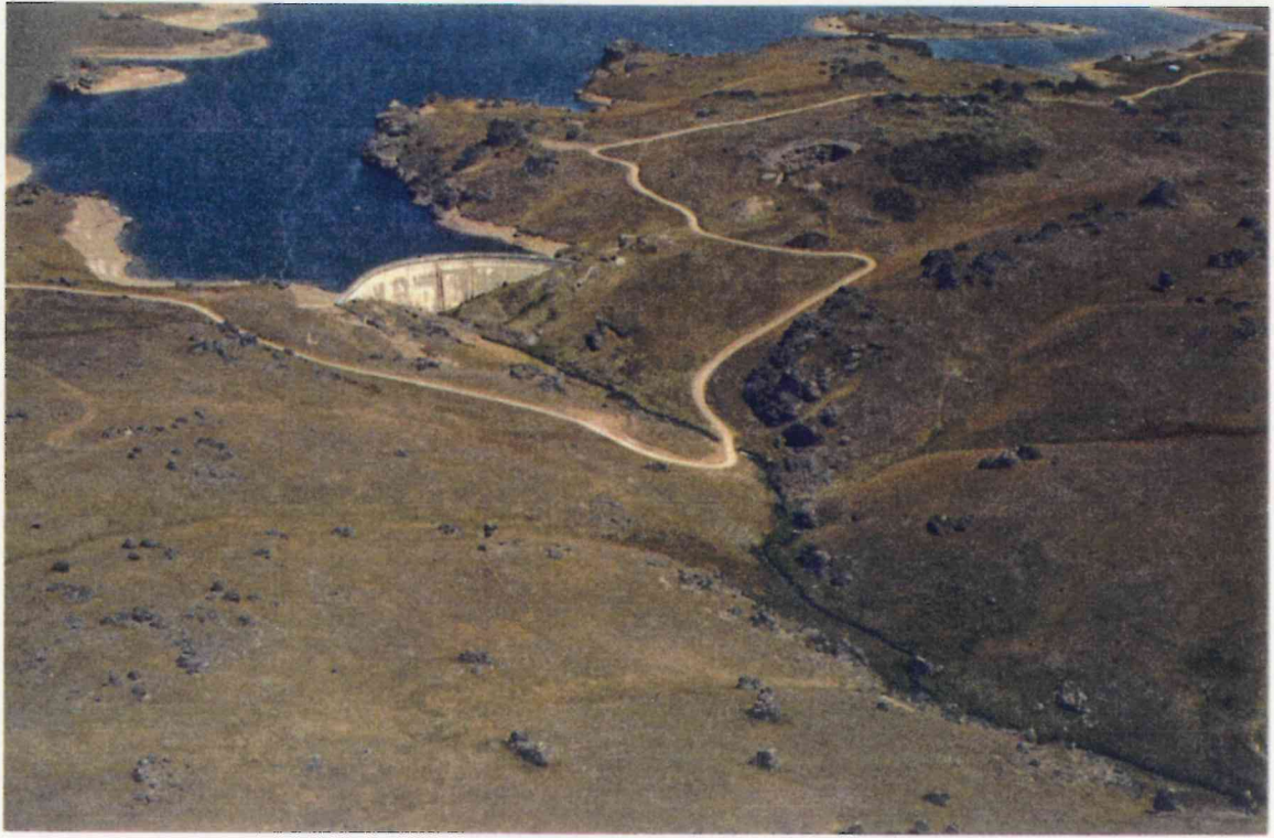
Poolburn Dam January 1990
