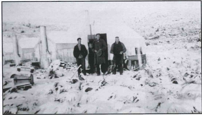
The timber framed canvas covered huts used by the PWD on construction works. Fireplaces at the end of the huts provided for warmth and cooking. This photo is not identified as being at Poolburn, but it illustrates the conditions that existed there.
