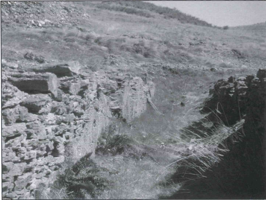
As it is today looking back up the recess for the covered conveyer used to bring stock-piled aggregate and sand to the mixing bins located at the concrete mixer. At the top left is the discarded stone from the crusher with the quarry above.
