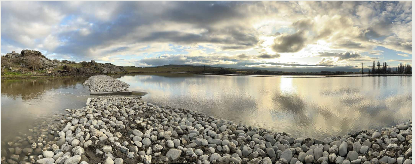
Wetland exit weir.
