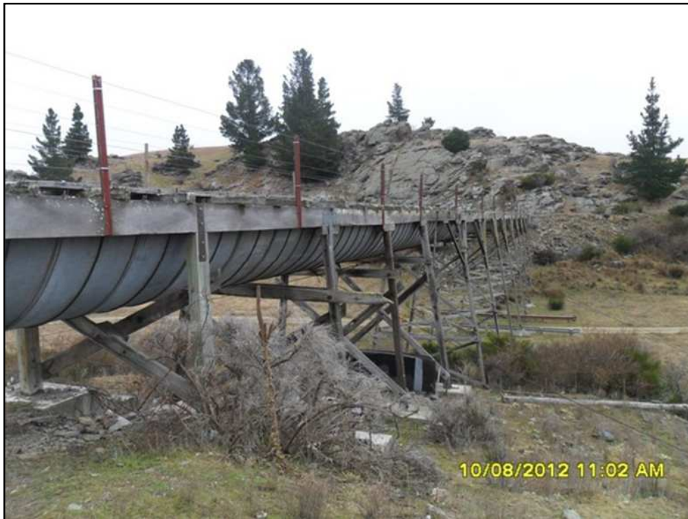
Figure 5: Chinky Gully Aqueduct
