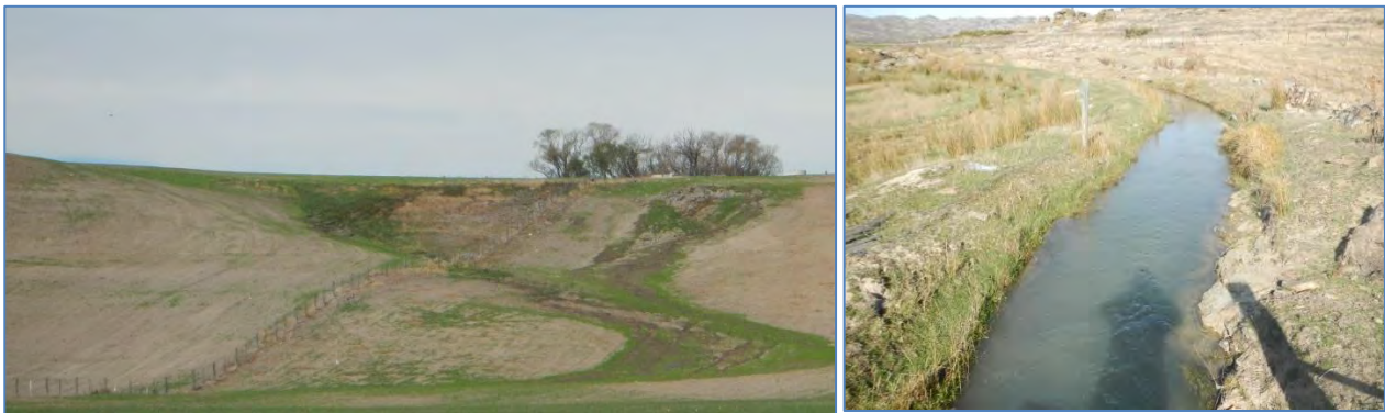
Figure 30: Omakau Irrigation Scheme photos indicating potential race leakage.
