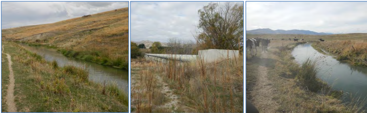
Figure 29: Omakau Irrigation Scheme typical races sections (left and right) and Becks Siphon (middle).
