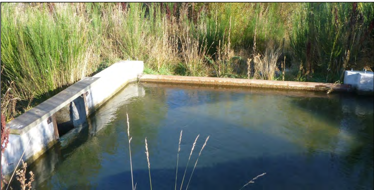
Figure 22: Blackstone Hill Irrigation Scheme Flow Control Weir.
