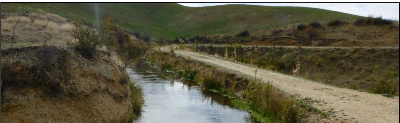
Figure 16: Manuherikia Scheme Main Race showing benching.
