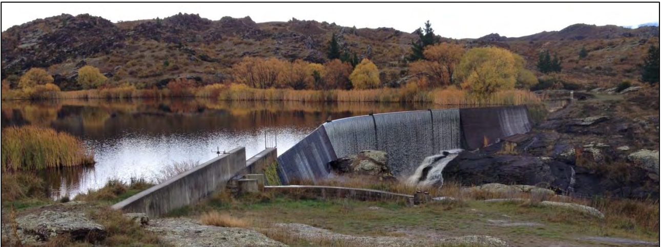
Figure 12: The Lower Manorburn Dam.
