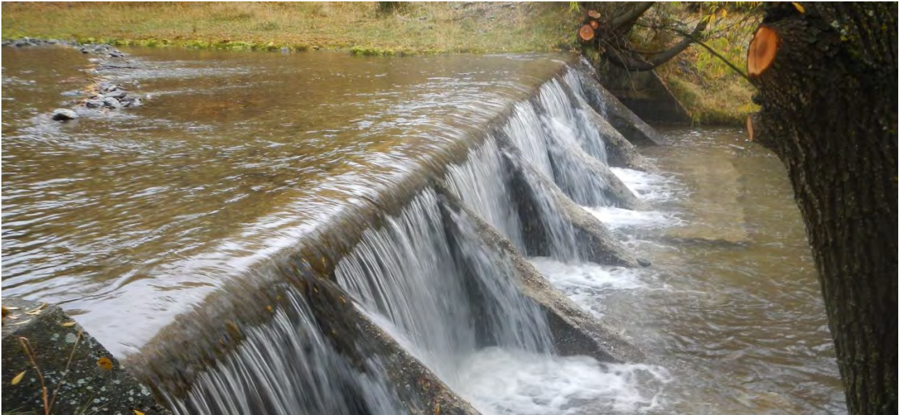
Figure 26: Omakau Irrigation Scheme – Lauder Creek weir.
