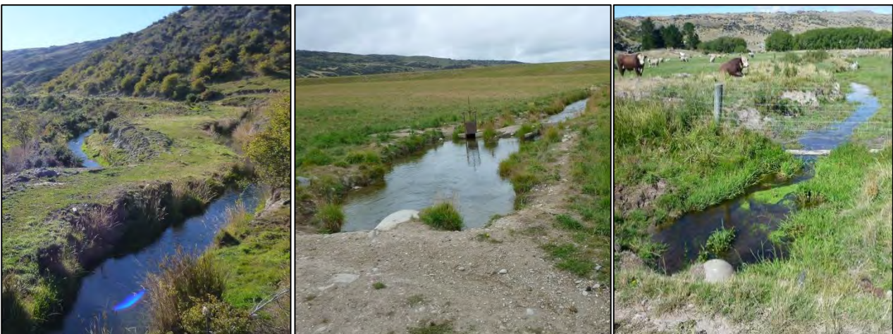
Figure 23: Blackstone Hill Irrigation Scheme: duel race section (left), typical race and farm crossing (middle) and race at Thurlow Road above bywash to Ida Burn (right).
