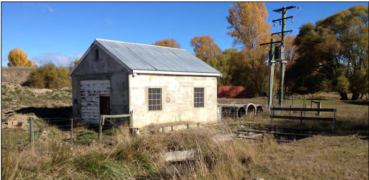
Figure 11: Galloway Irrigation Scheme Manuherikia pump station.
