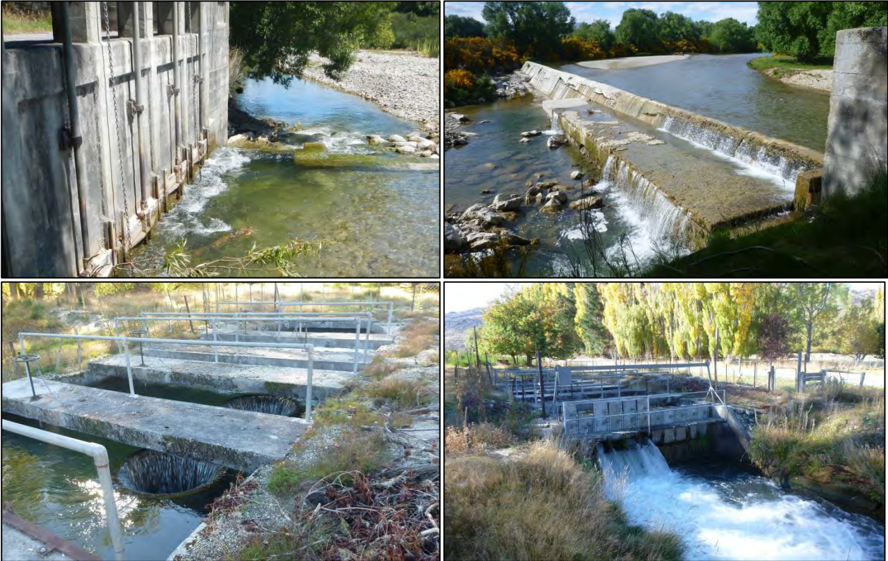
Figure 24: Omakau Irrigation Scheme - Main Race intake weir and flow control structure.
