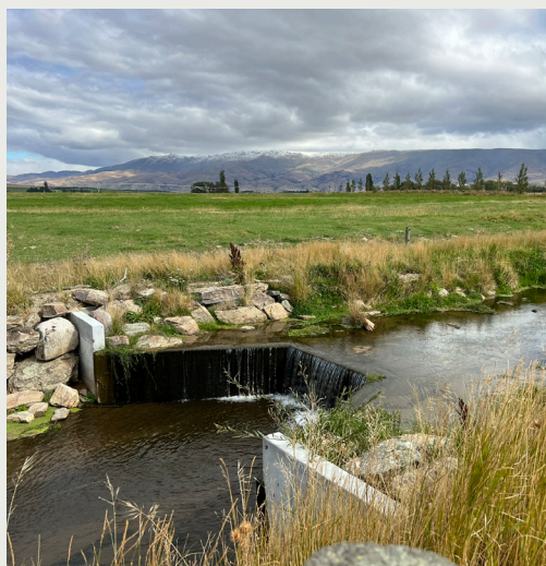
Photo Source: Fish barrier installed in Thomsons Creek
