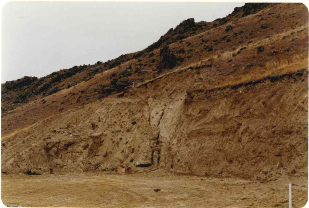
Plate 13 Tension Cracks in the borrow pit (The core boxes give scale)
