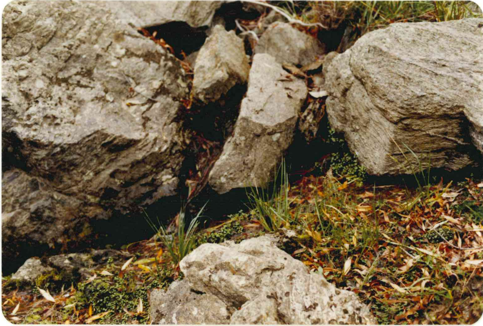
Plate 12 Water Seep from Buried Pipe Landslide RS 436-515
