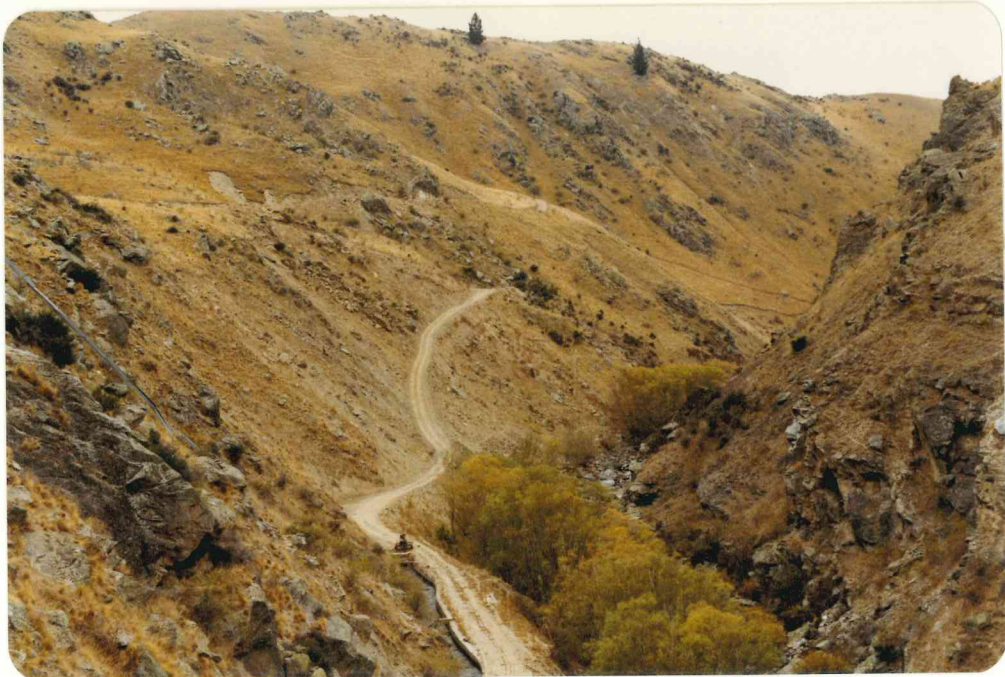
Plates 9, 10 & 11 Landslide at RS436-515
