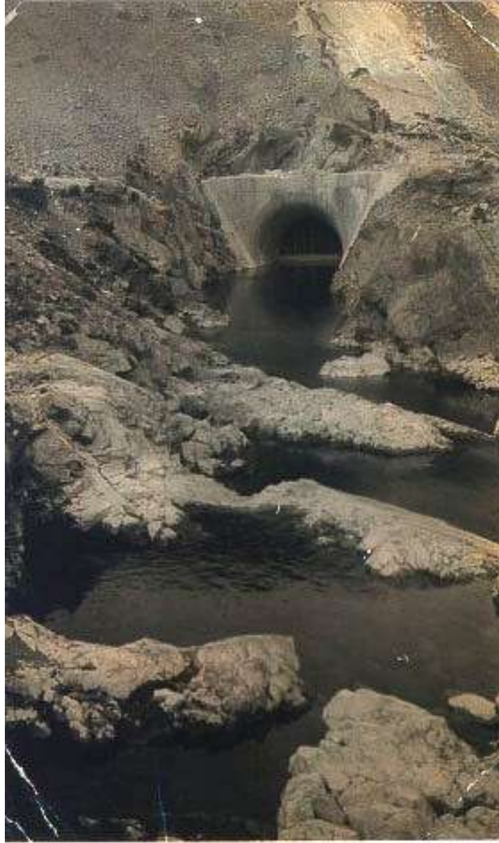
Figure 9 Left abutment diversion tunnel
