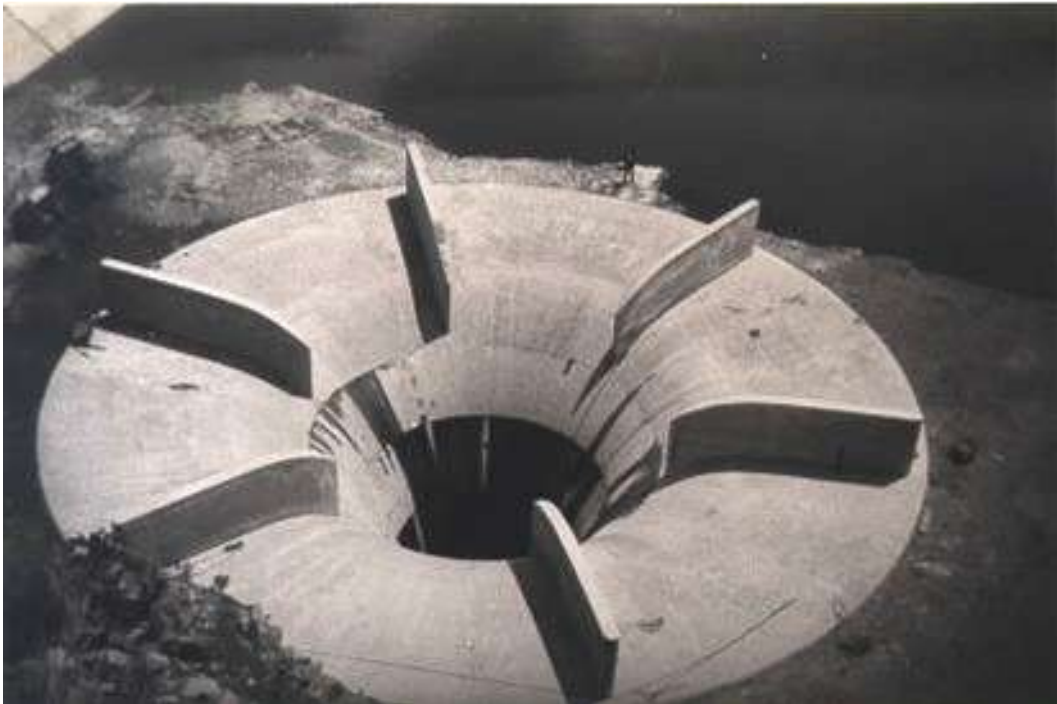
Figure 10 Morning Glory Spillway Construction
