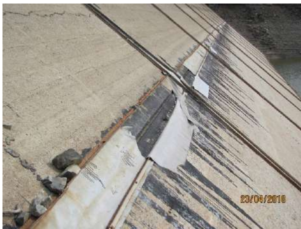
Figure 25 (a) & (b) Joint repair condition
