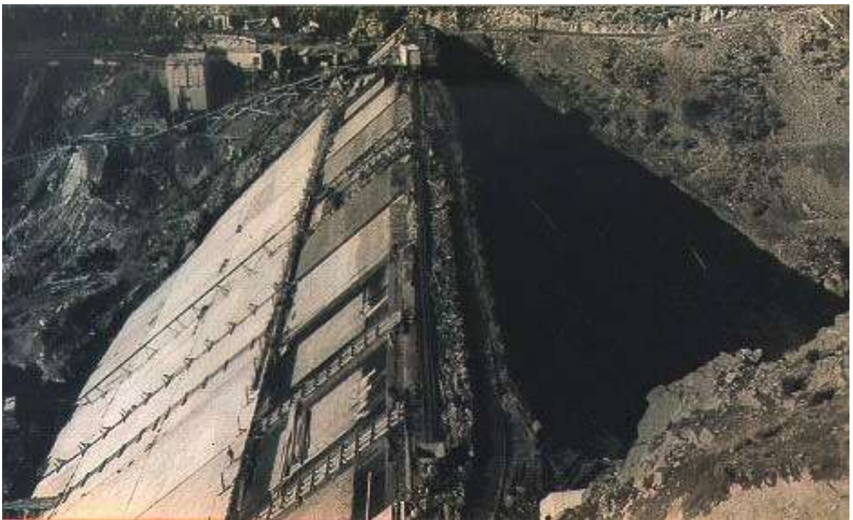
Figure 14 Concrete facing nearing completion
