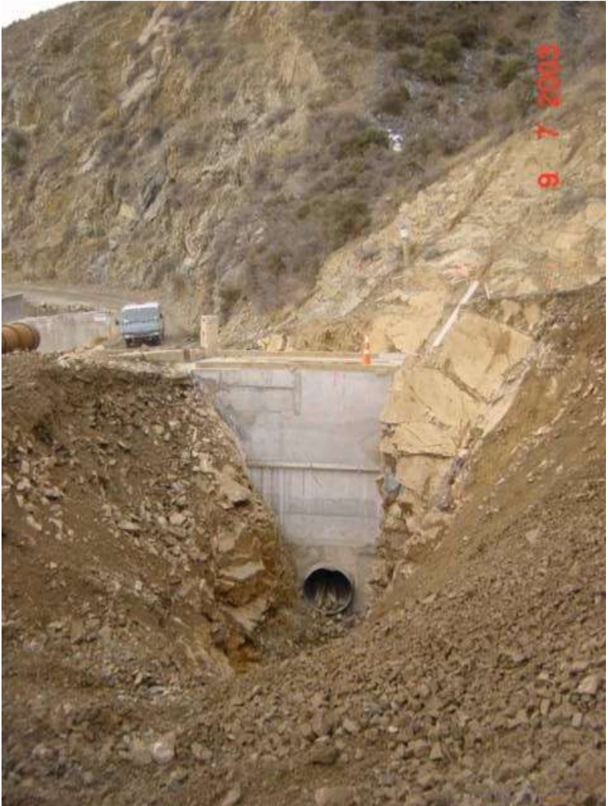
Figure 19 Syphonic penstock penetration through extended cut off
