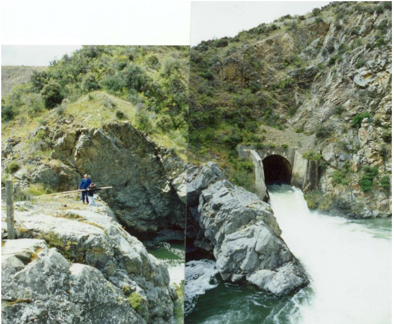
Figure 11 Tunnel outlet c2002 prior to hydropower scheme development
