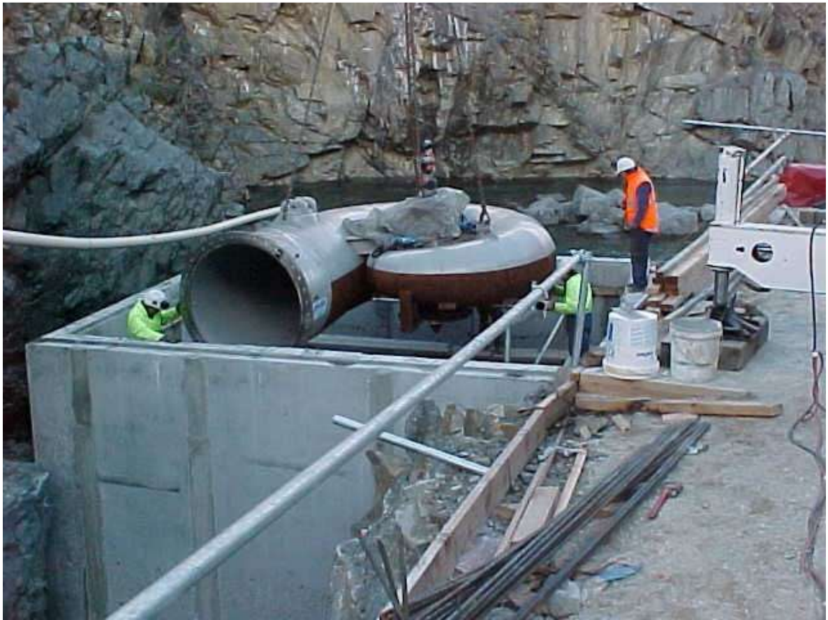
Figure 20 Tanked powerhouse construction at the “falls”
