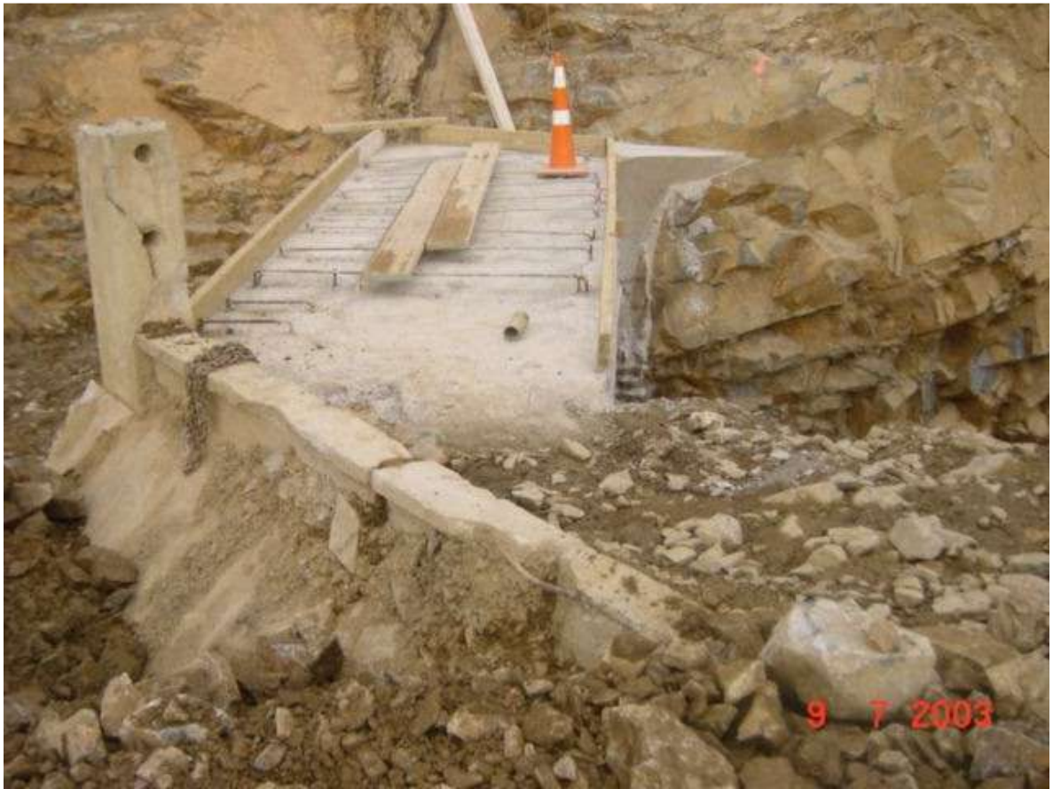
Figure 18 Extension to plinth cut off trench at left abutment crest
