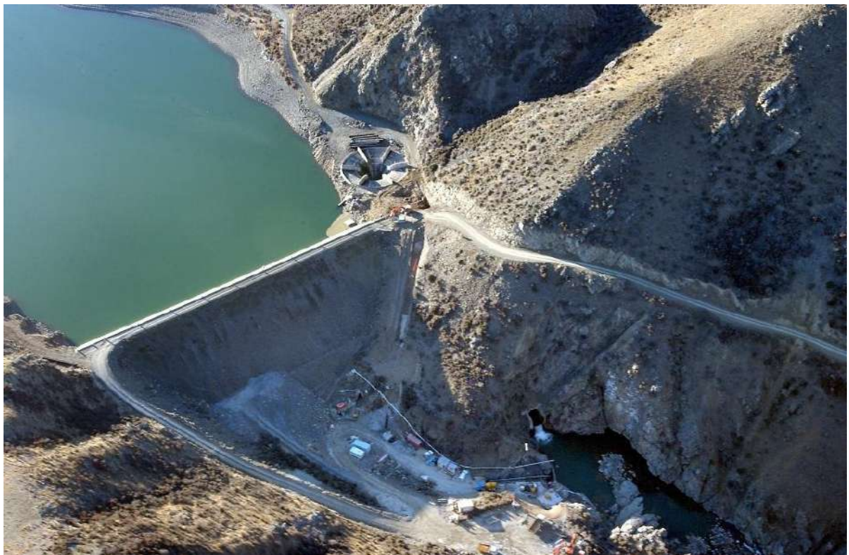
Figure 22 Aerial view of hydropower scheme construction
