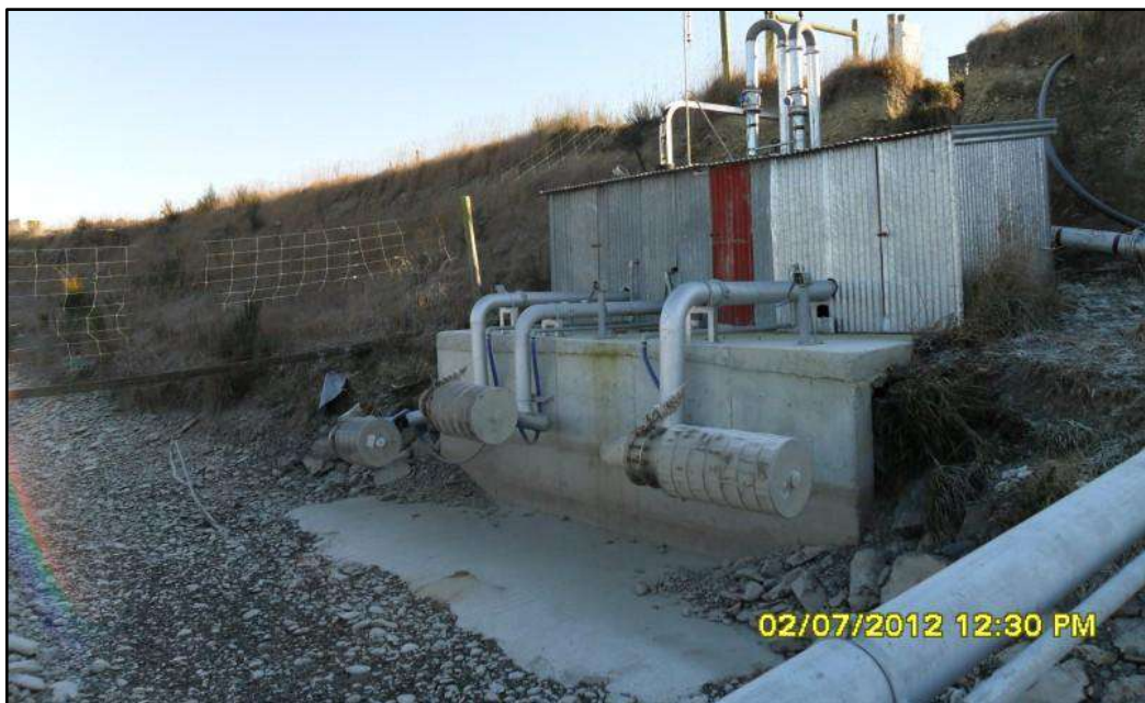
Figure 25: Example of pumping from a race
