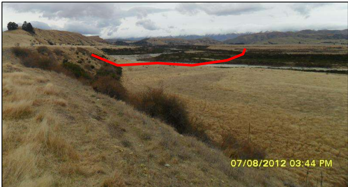
Figure 20: Manuherikia siphon (looking east)
