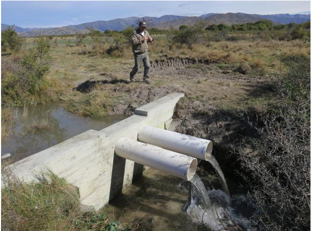
Figure 16 A built barrier designed to prevent salmonid incursion in Omarama spring. Credit Dean Nelson
