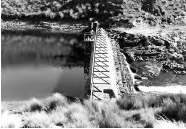
Figure 19. Lake Onslow Dam 1971
