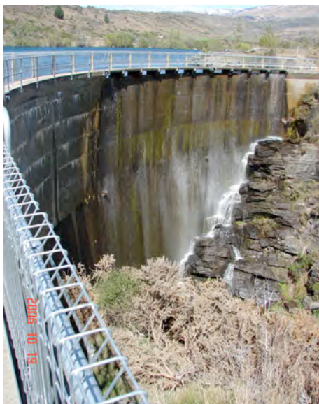
Figure 22. Conroys Dam from right bank
