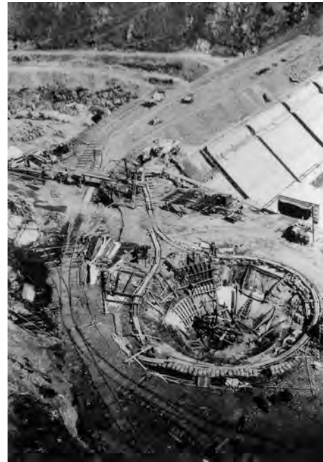
Figure 20. Falls Dam under construction 1934 showing morning glory spillway in foreground
