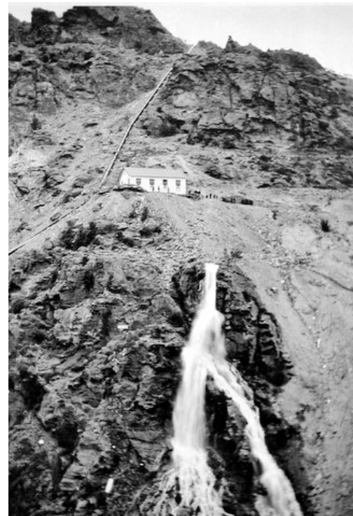
Figure 17. Original Teviot (George) power station
