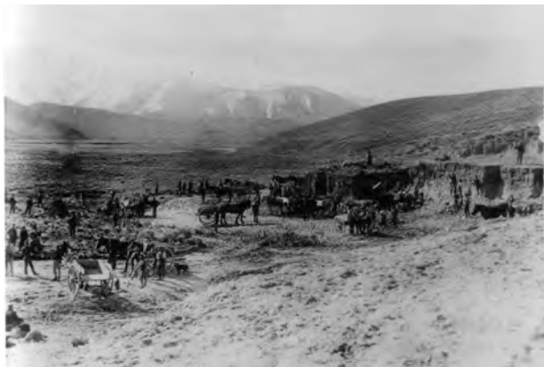
Figure 2. West Eweburn Dam construction 1898?
