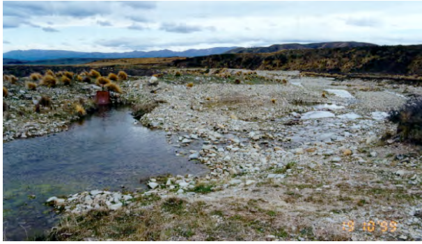
Figure 5. Hills Creek intake
