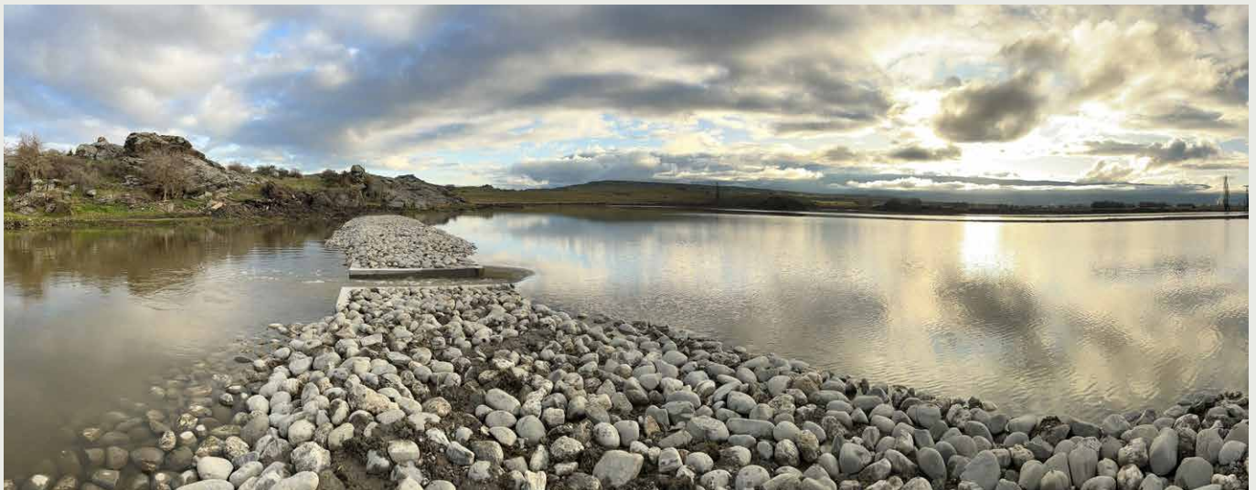
View of the completed exit weir.
